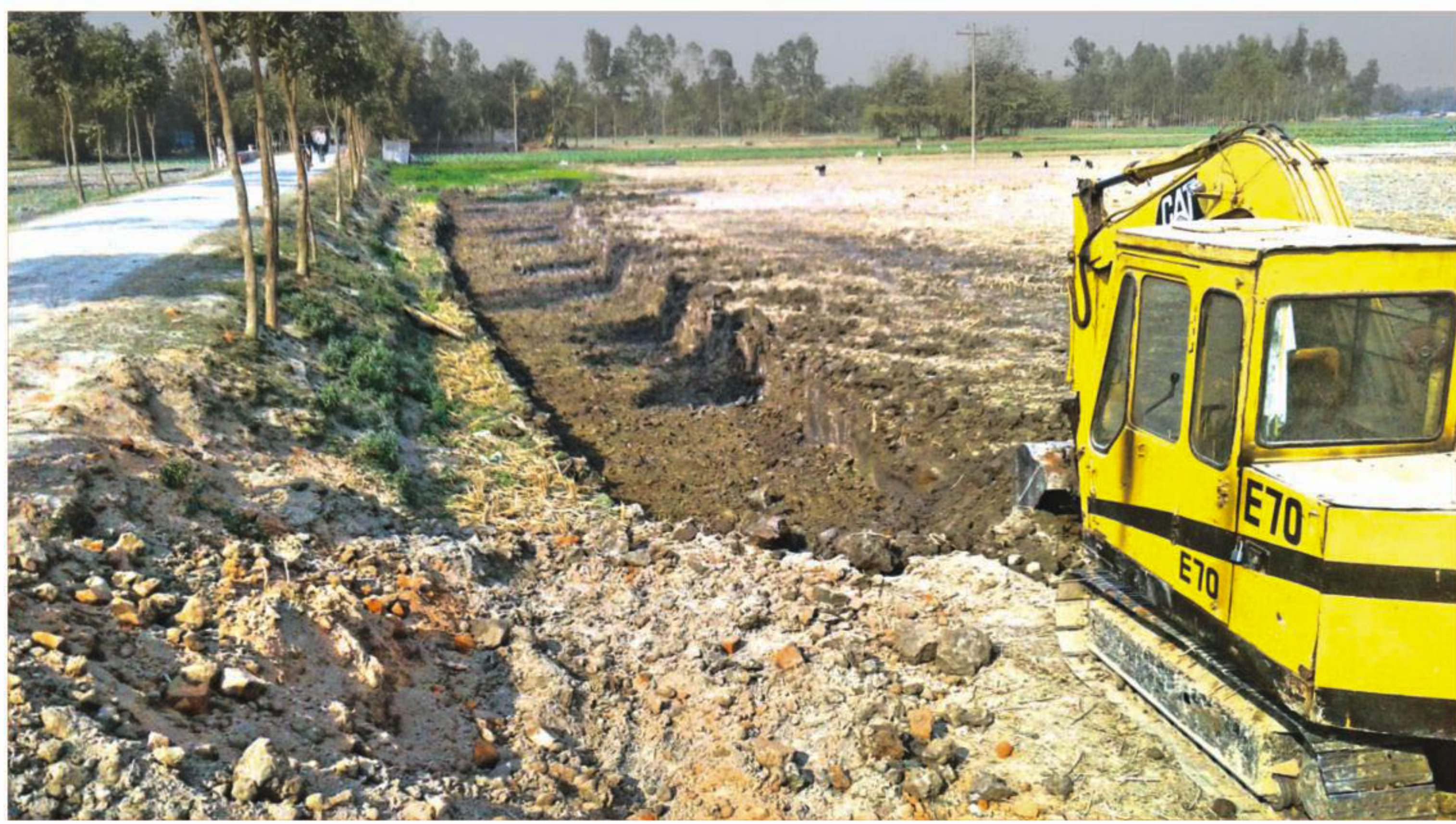
Many such village roads in Lalmonirhat are facing threat of collapse as influential brick kiln owners continue removing the topsoil from roadside farmlands, using excavator machines. The photo was taken from Devirpat village in Aditmari upazila recently.
