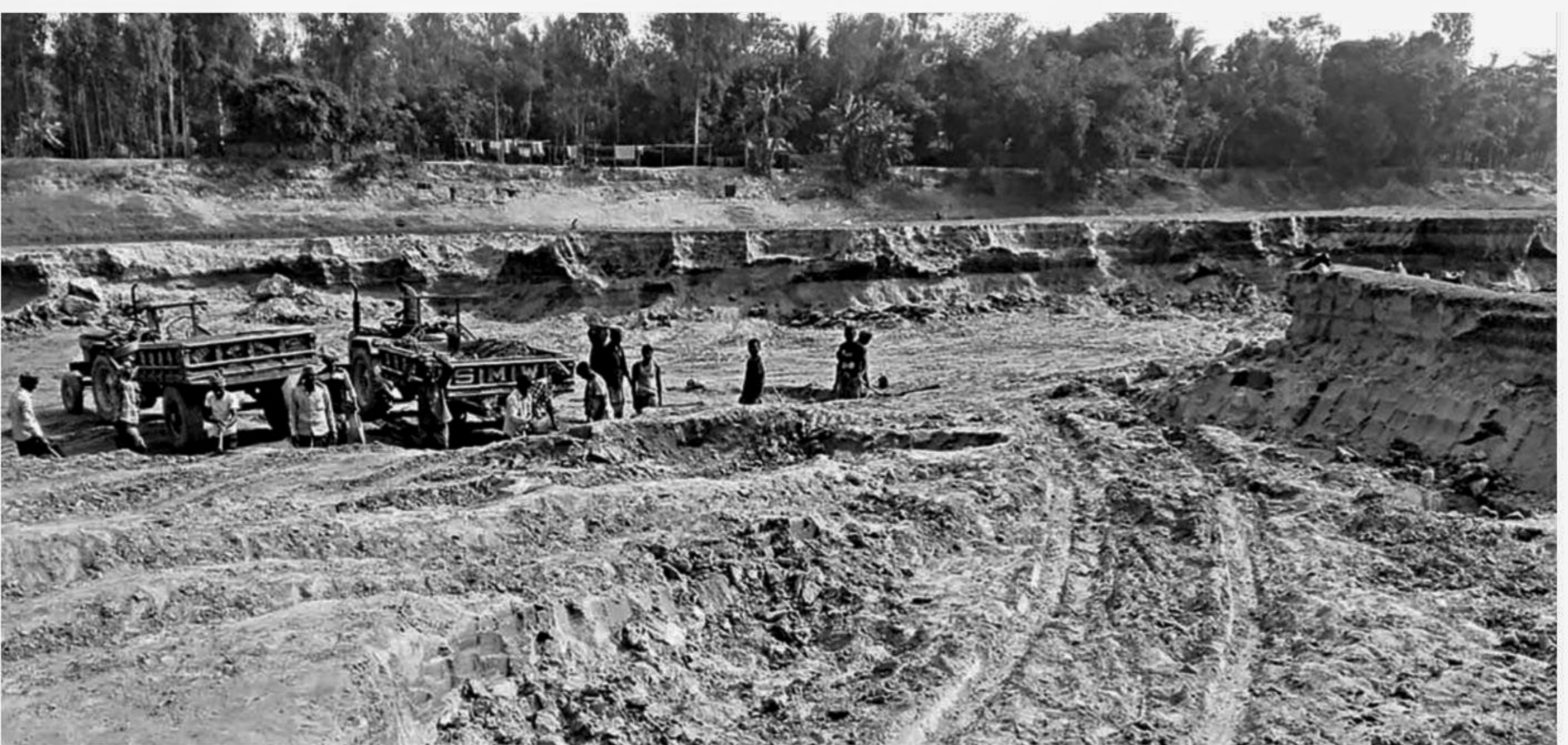
Unabated earth lifting from the Ghagot riverbed threatens the town protection embankment at Karmonai in Kholahati union of Gaibandha.
