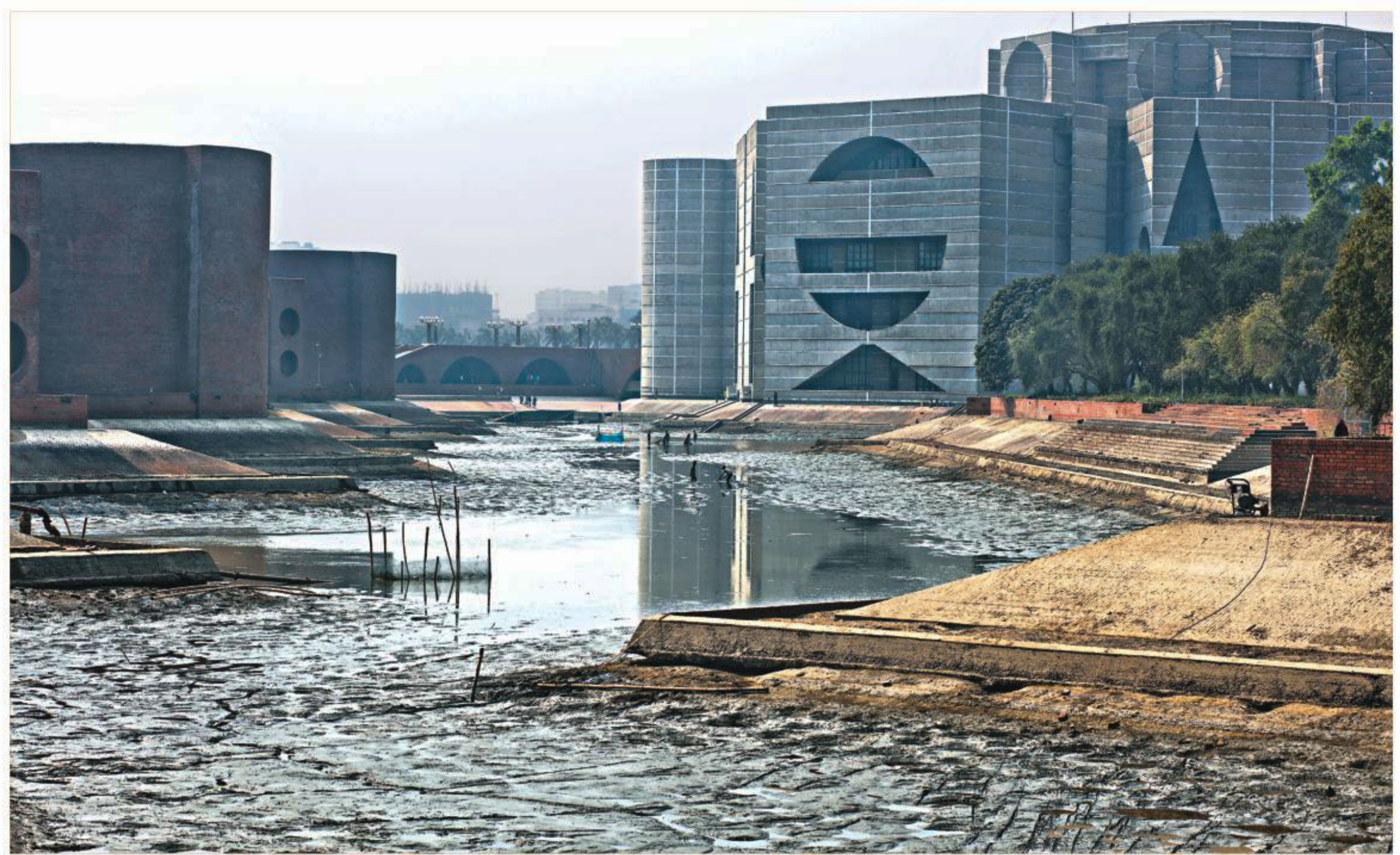
Water being drained out from the lake surrounding Sangsad Bhaban, to clear the layer of mud underneath and check for cracks on the concrete lake floor, as part of a restoration project. The photo was taken yesterday.
