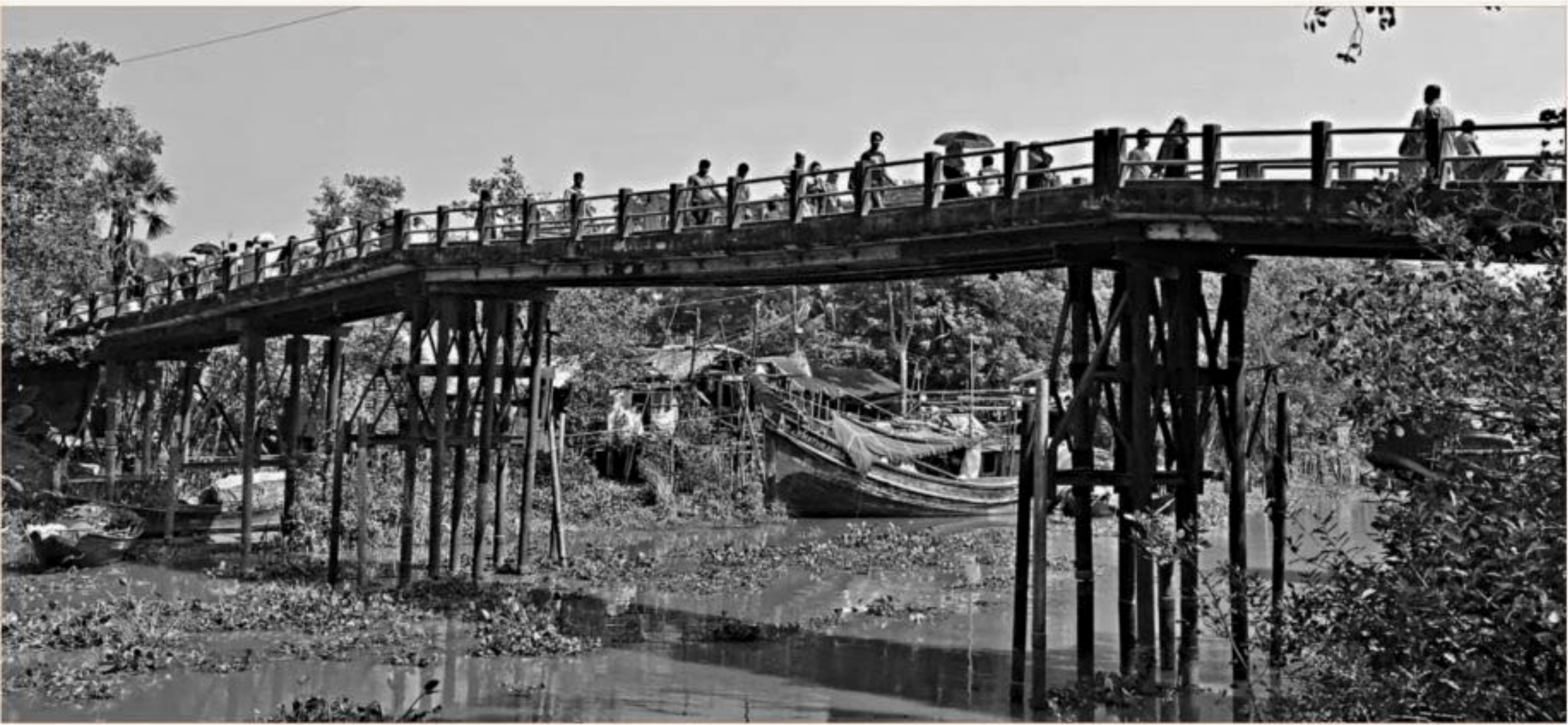
People cross the risky bridge on the Rayenda river at Rayenda Bazar in Bagerhat's Sharankhola upazila. Iron pillars of the structure are badly damaged.
