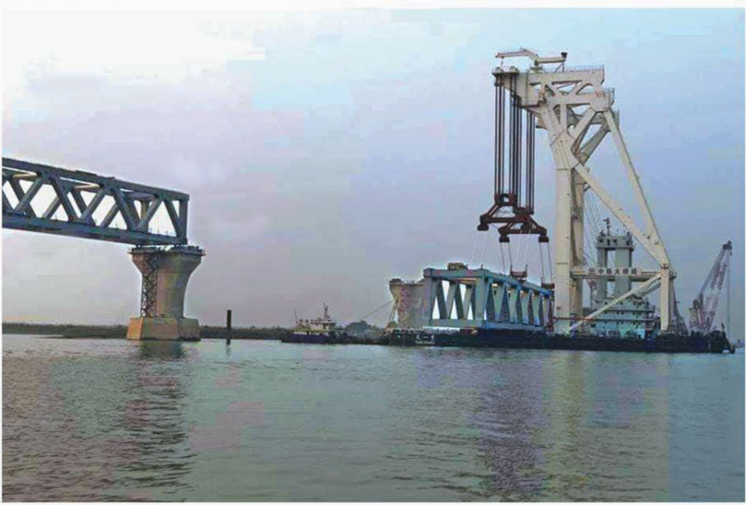
The sixth span of the Padma Bridge has been brought to near pear-36 at Jazira point of Shariatpur. The 150-metre-long superstructure is likely to be placed between pear-36 and 37 today. Following its placement, 900 metres of the 6.15 km bridge will be visible. The photo was taken yesterday.
