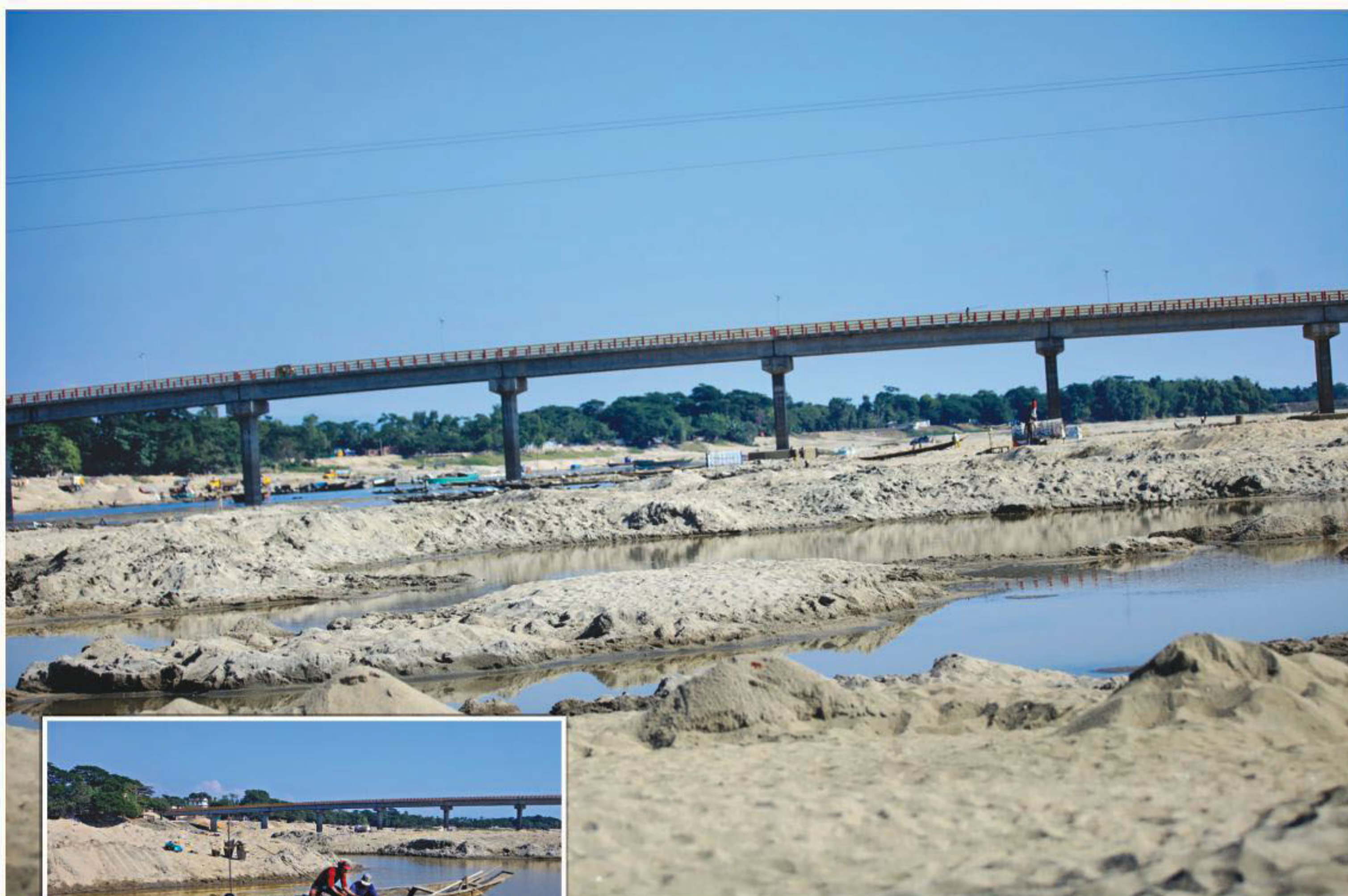
Illegal sand and stone extraction on the Piya river bed has altered the landscape of Jafong in Sylhet's Gowainghat. The gaping holes near the bridge, which was open to traffic last year, may weaken its pillars. Inset, villagers extract stones from the river. The picture was taken recently.
