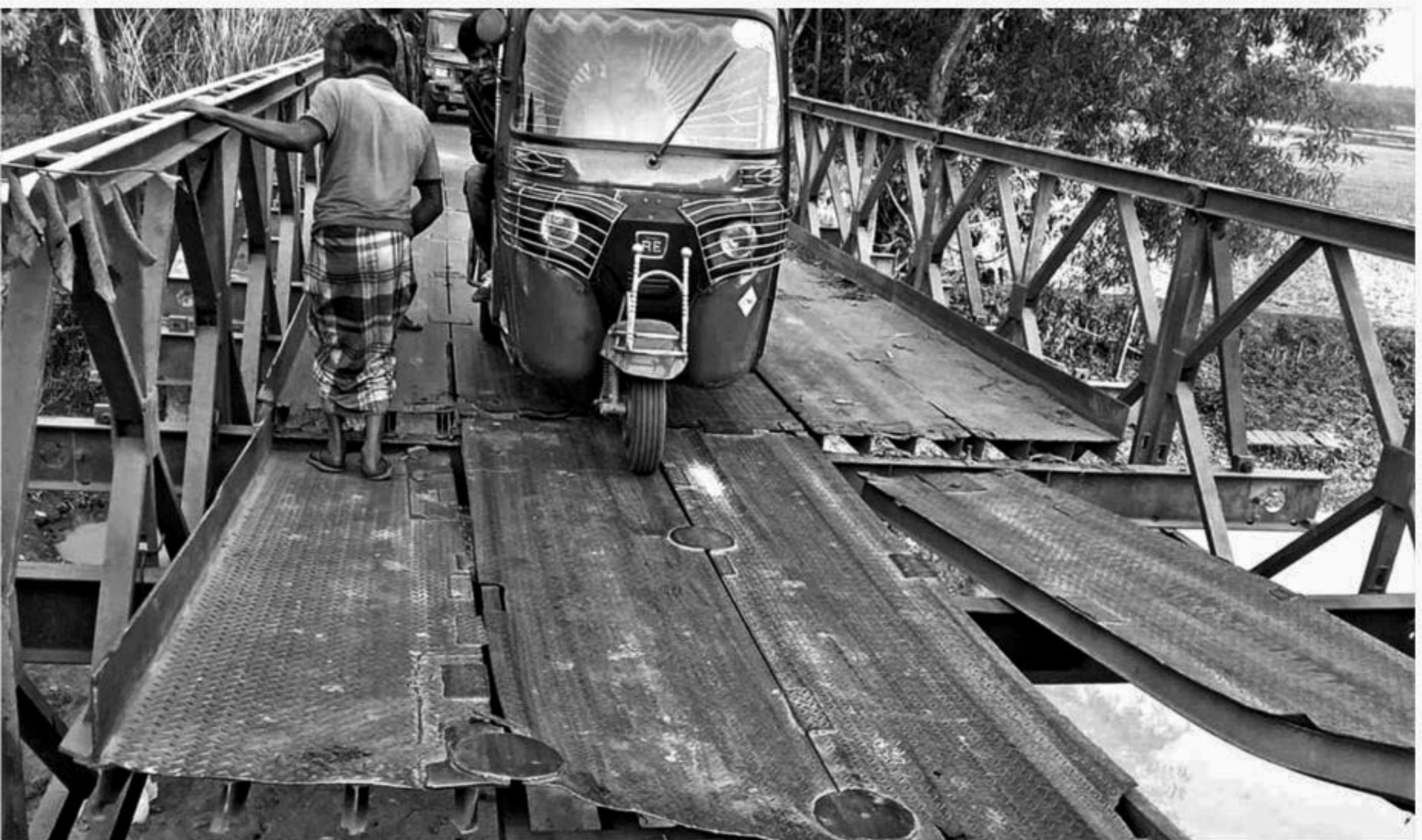
This Bailey bridge on Sakhipur-Batajore road at Kirtonkhola Dhumkhali in Sakhipur upazila of Tangail has remained in an awful condition after it got badly damaged under the pressure of a loaded truck on December 29.
