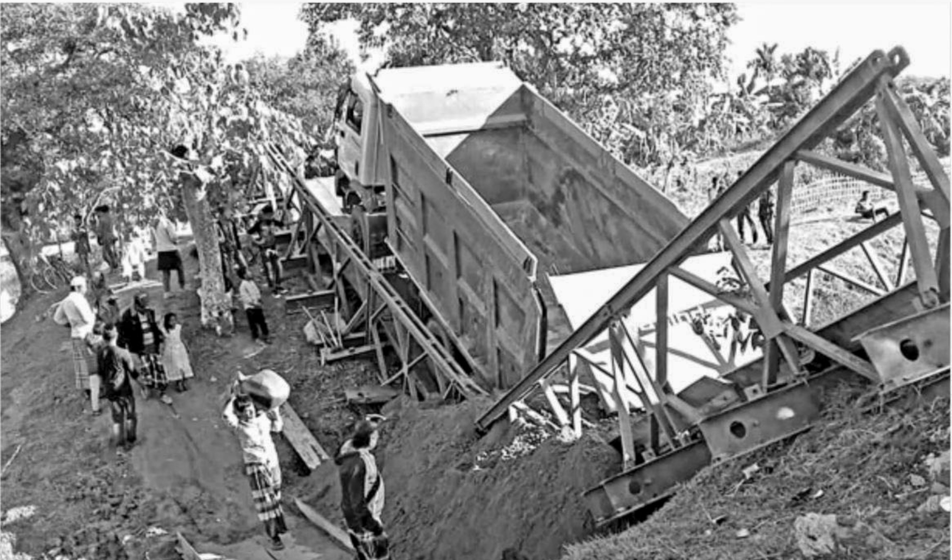
An overloaded truck gets stuck as the Bailey bridge over Ratura canal in Moulvibazar's Juri upazila broke down due to the pressure of the vehicle on Friday.
