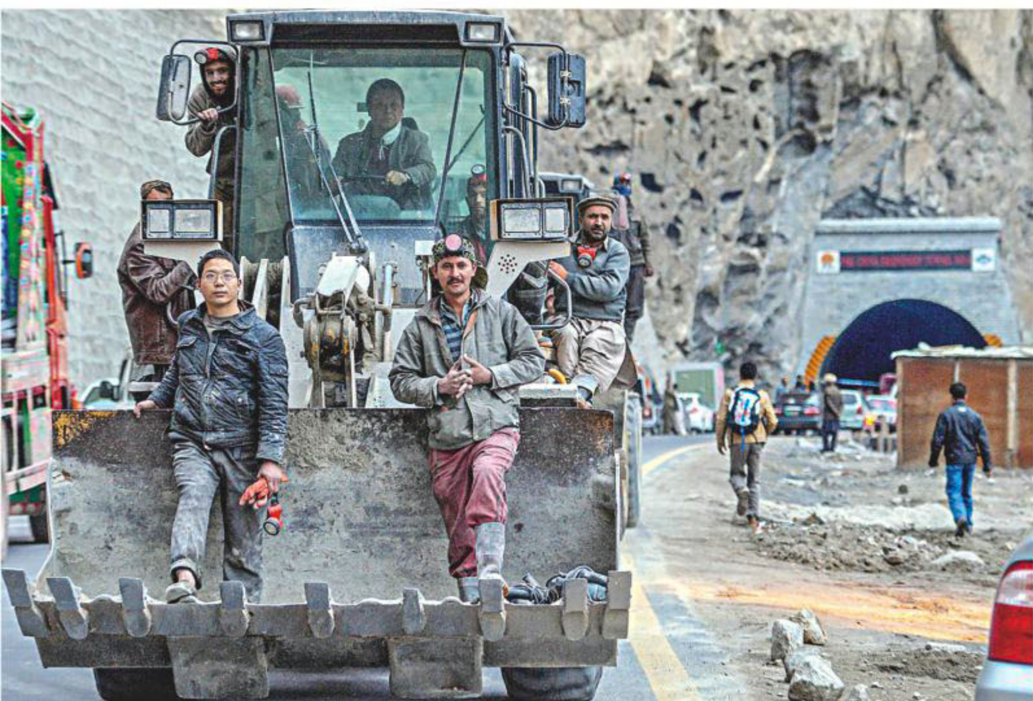
Chinese and Pakistani workers sit on an excavator as they leave a newly built tunnel in northern Pakistan.
