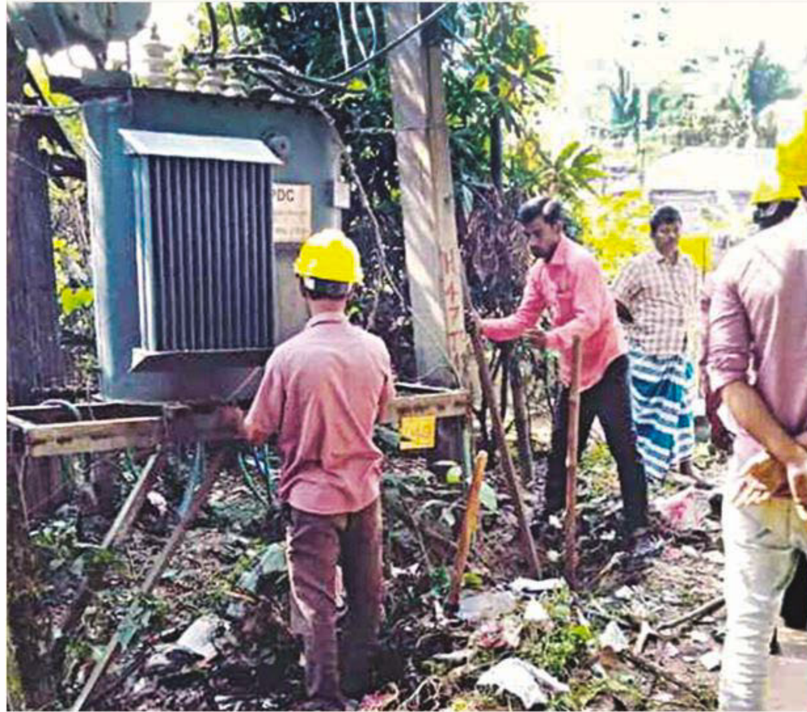
Employees of Dhaka Power Distribution Company shifting a transformer to a higher place in the capital's Nasirabad yesterday, a day after The Daily Star ran a photo, right, showing that the transformer was barely two feet above the ground, posing risk to locals, especially children.
