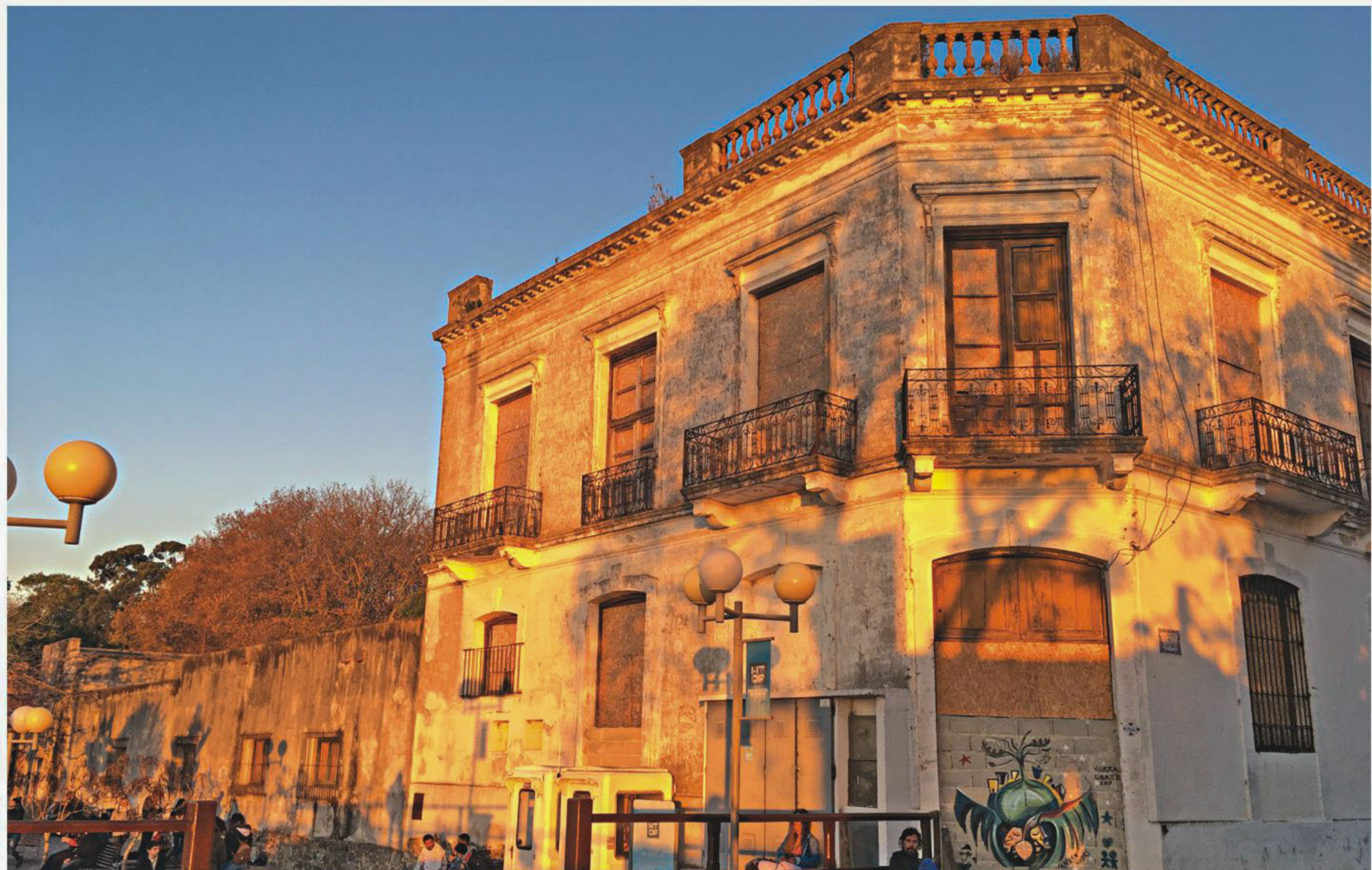
The setting sun casts an orange glow over crumbling buildings
