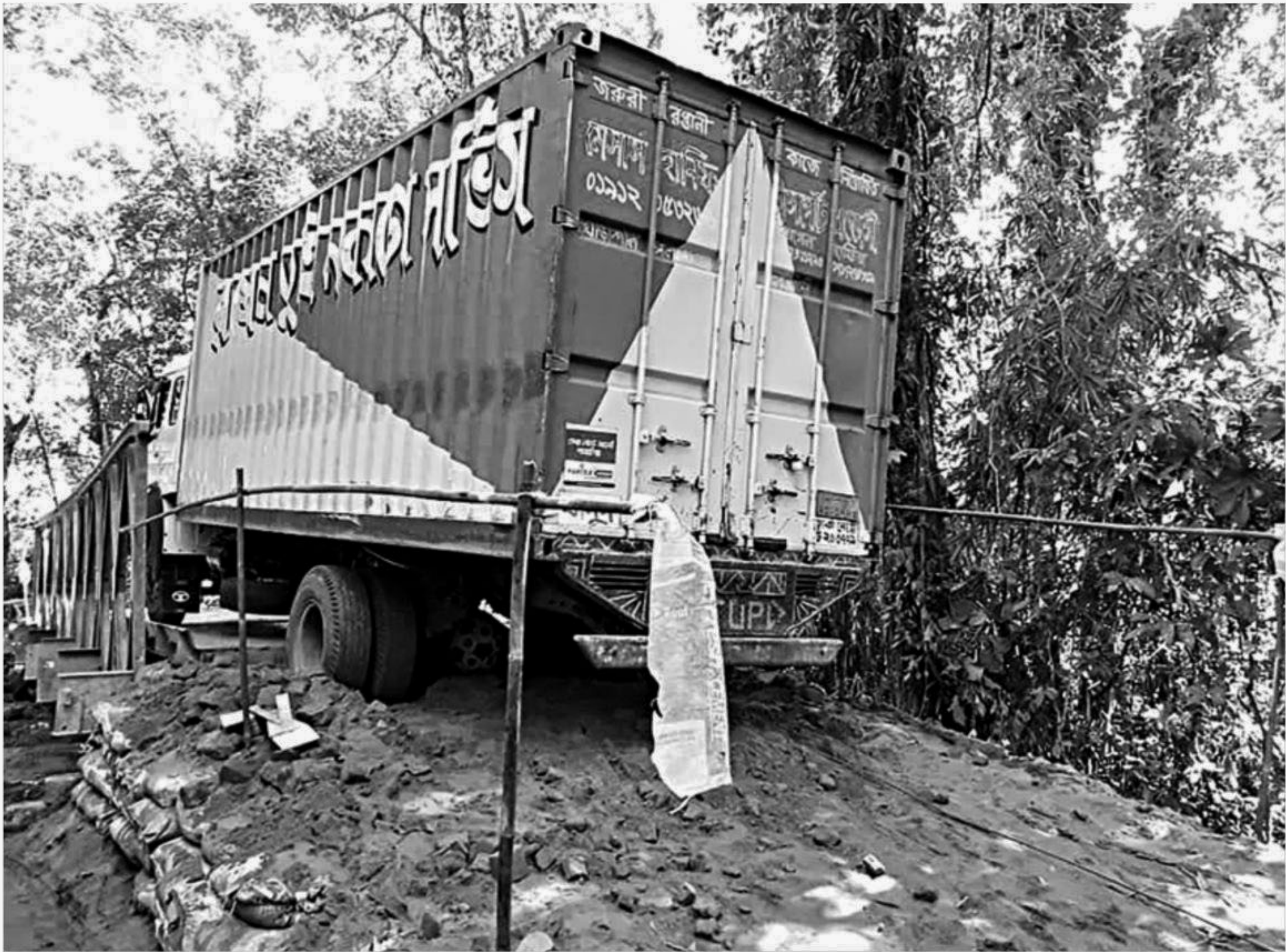
This Bailey bridge in Lawacherra forest area of Sreemangal upazila in Moulvibazar caved in under the pressure of a coal-laden truck early Thursday. Road communication with adjacent Kamalganj upazila remained suspended since then as the repair work could not be complete as of yesterday evening.
