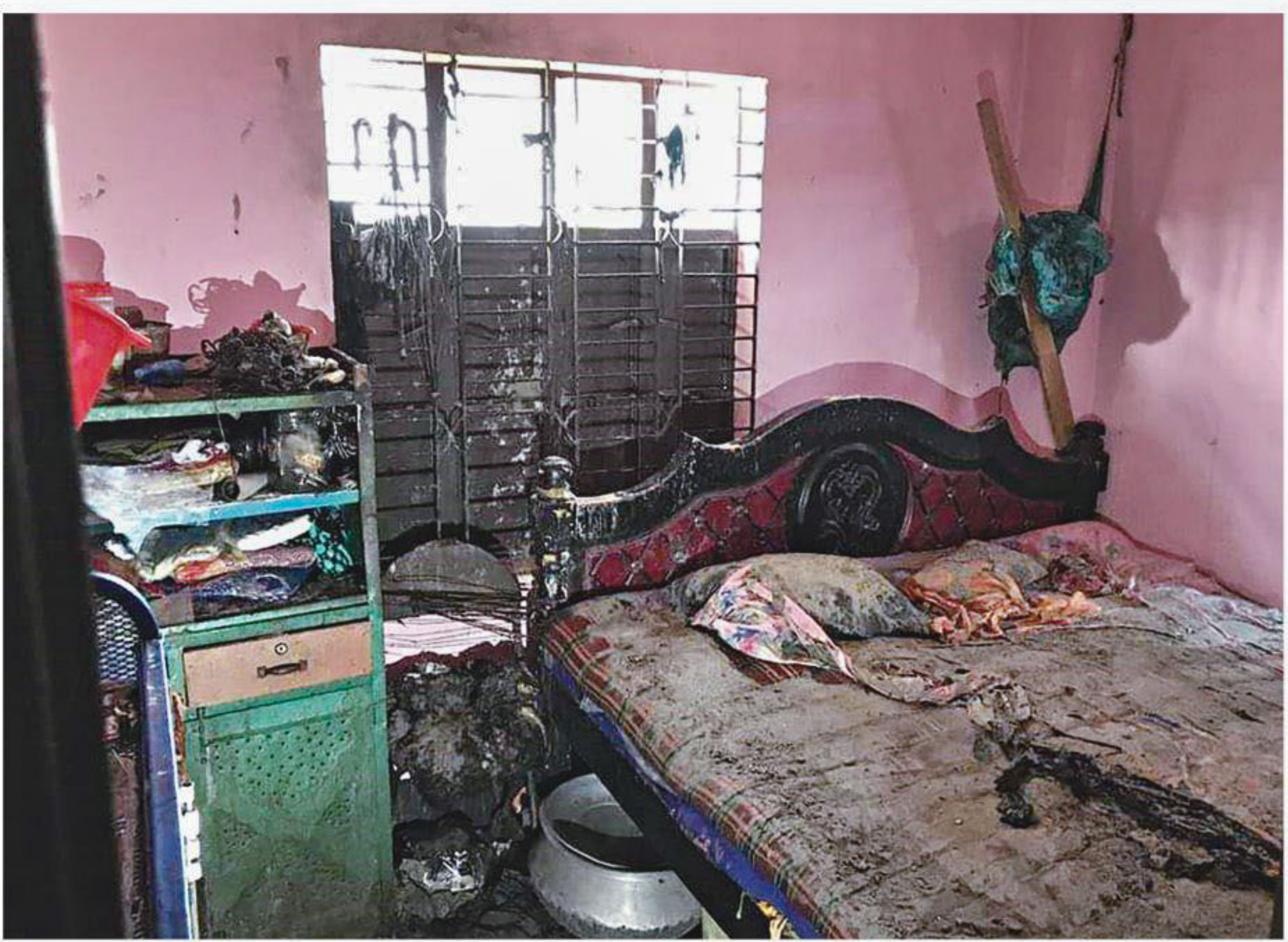
A room of the flat in Ashulia where five members of a family suffered burns in an explosion caused possibly by a gas line leak yesterday.
