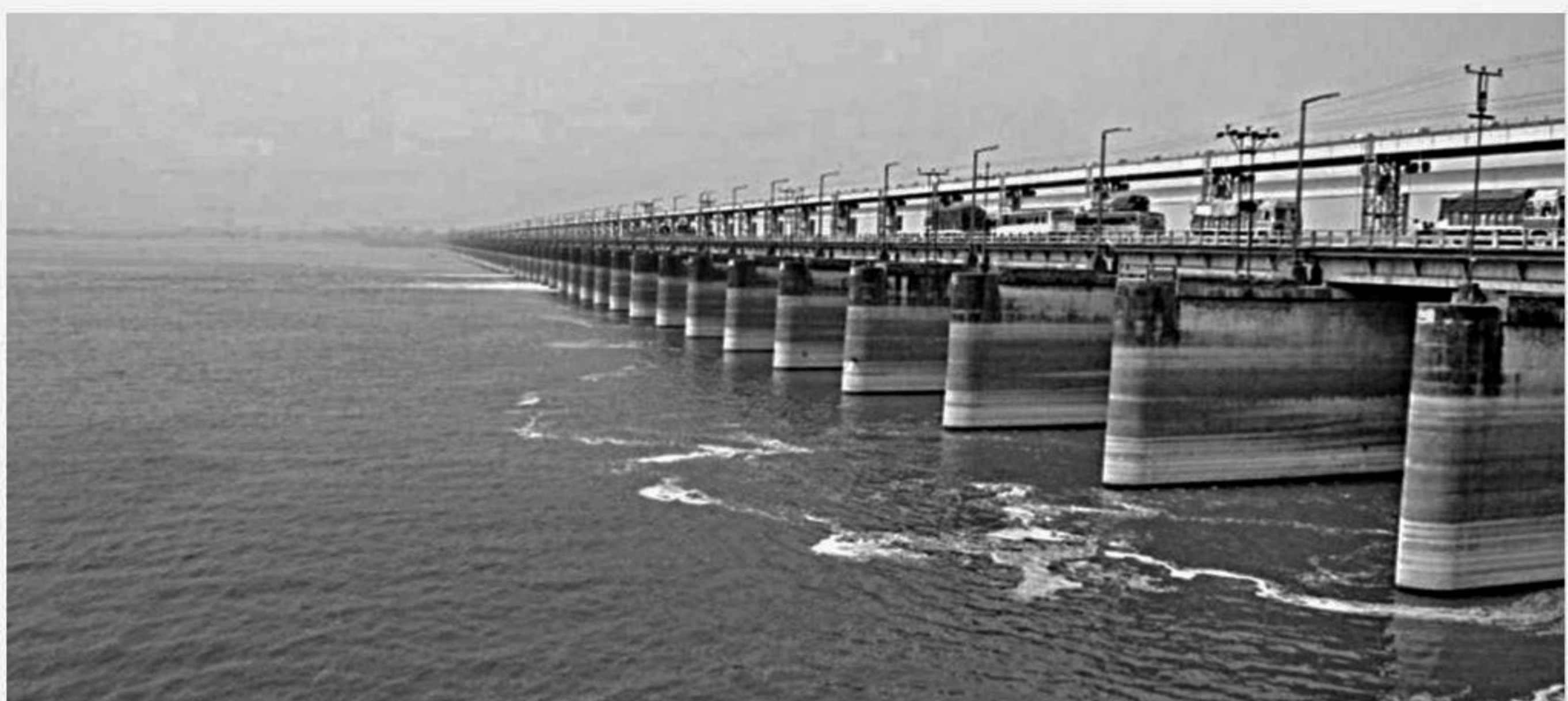
Farakka Barrage across the Ganges River.
