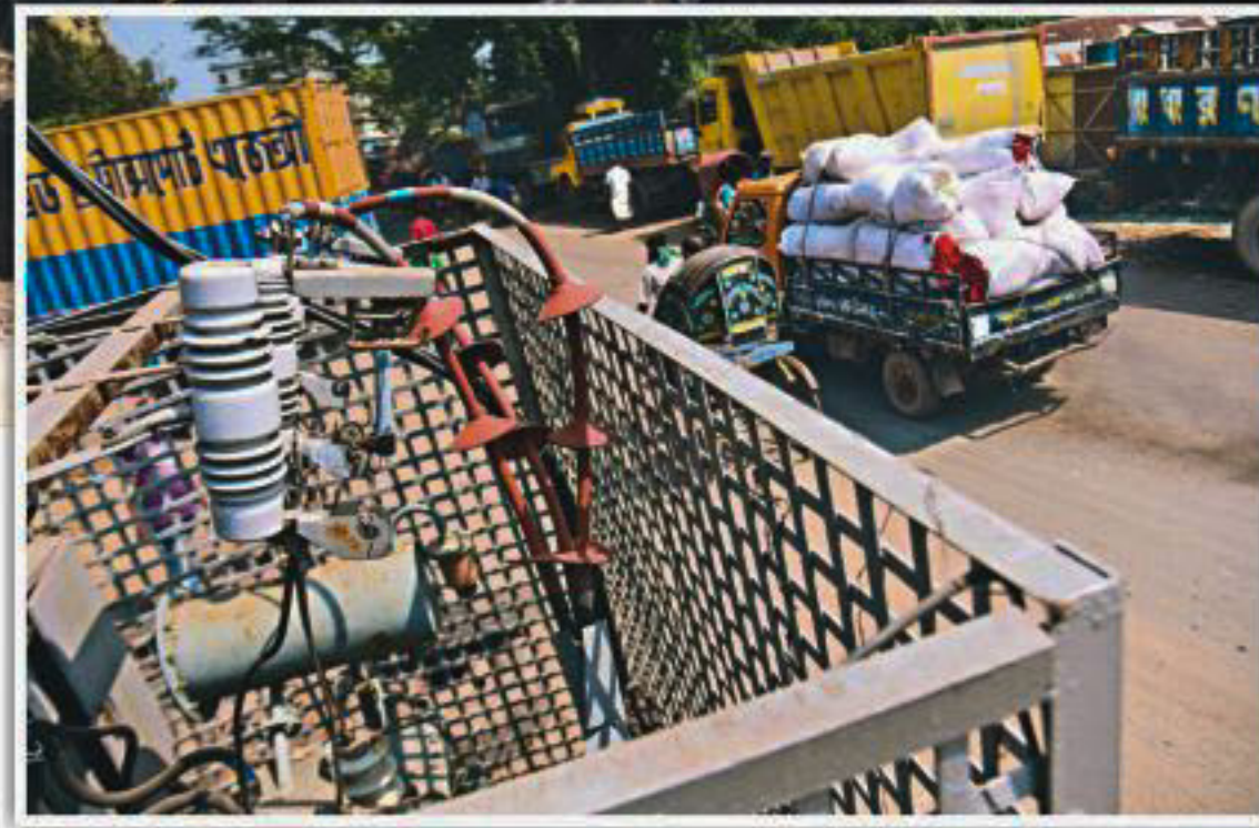
A man walking by a high-voltage transformer, kept inside a cage, in Majhirhat area of Chattogram city yesterday. The transformer, which is set on a trolley, is also occupying part of the road. According to locals, it was set up temporarily around five months ago after the existing one went out of order. As per rule, such a transformer is to be set on electric poles with special protective arrangements to avoid any accident.
