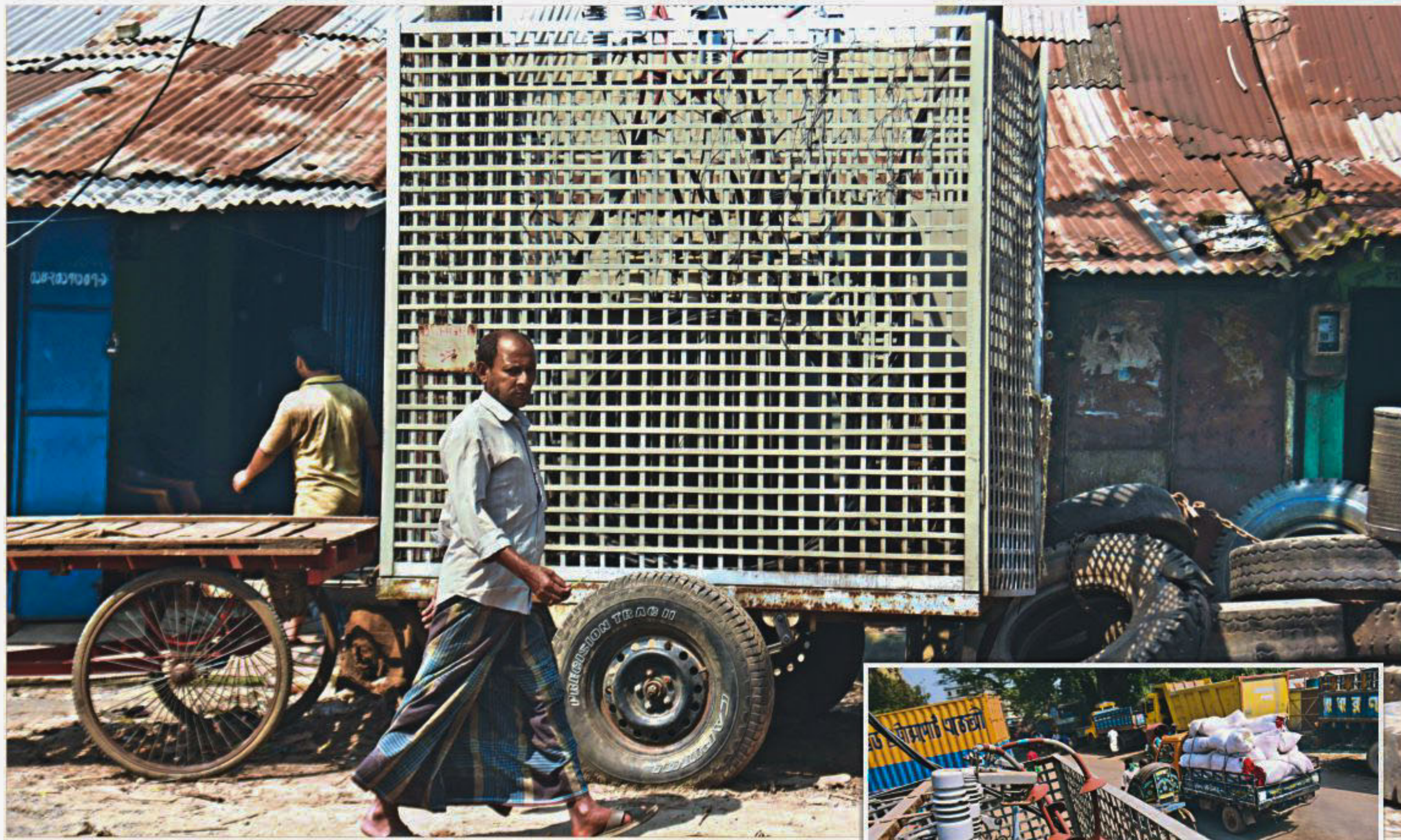
A man walking by a high-voltage transformer, kept inside a cage, in Majhirhat area of Chattogram city yesterday. The transformer, which is set on a trolley, is also occupying part of the road. According to locals, it was set up temporarily around five months ago after the existing one went out of order. As per rule, such a transformer is to be set on electric poles with special protective arrangements to avoid any accident.
