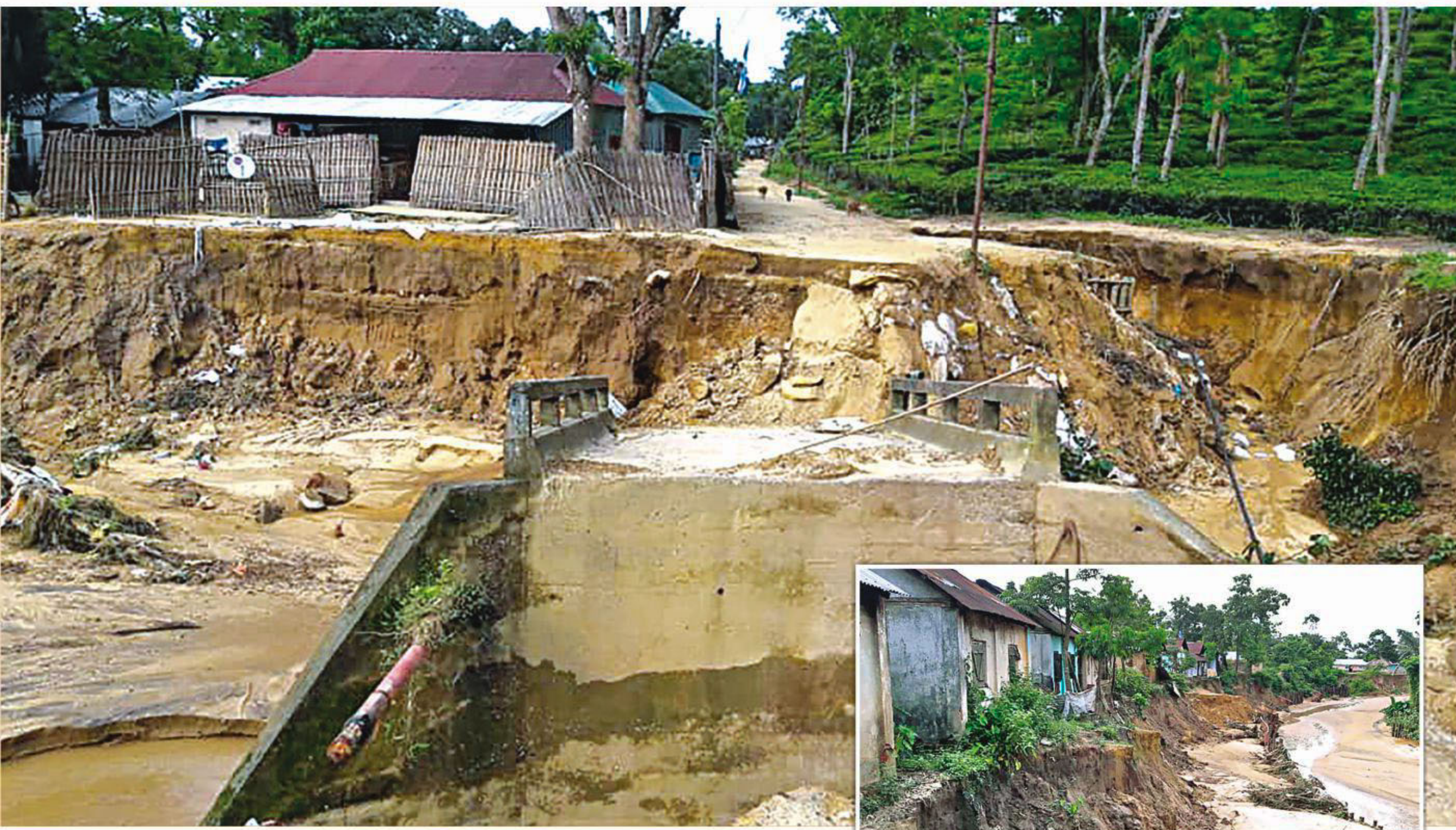
This concrete bridge along with a portion of the bridge approach road collapsed in June this year due to illegal lifting of sand from a canal flowing along a tea garden in Habiganj's Chunarughat upazila. Inset, mindless sand lifting has eroded 40 such houses at Chaklapunjee Tea Garden.
