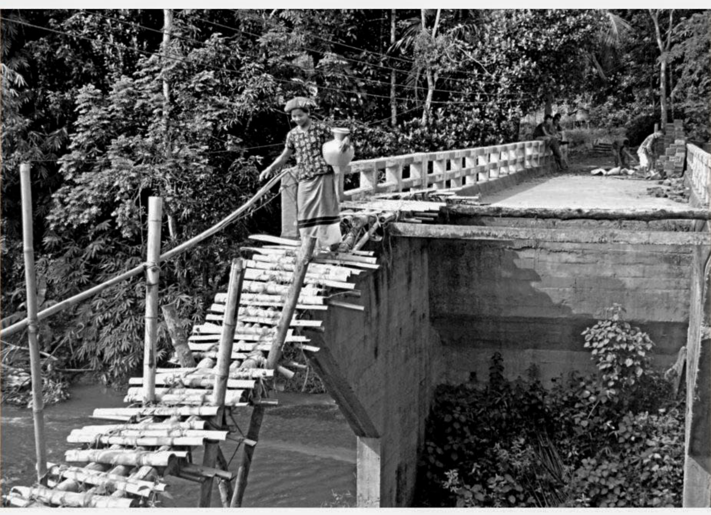
The bridge at Dewanpara village in Kawkhali upazila of Rangamati lies without repair after its partial collapse during last year's flood. Right, people cross risky bamboo bridges at Ananda Bazar in Faridpur Sadar upazila and Barobazar union in Kaliganj upazila of Jhenidah.
