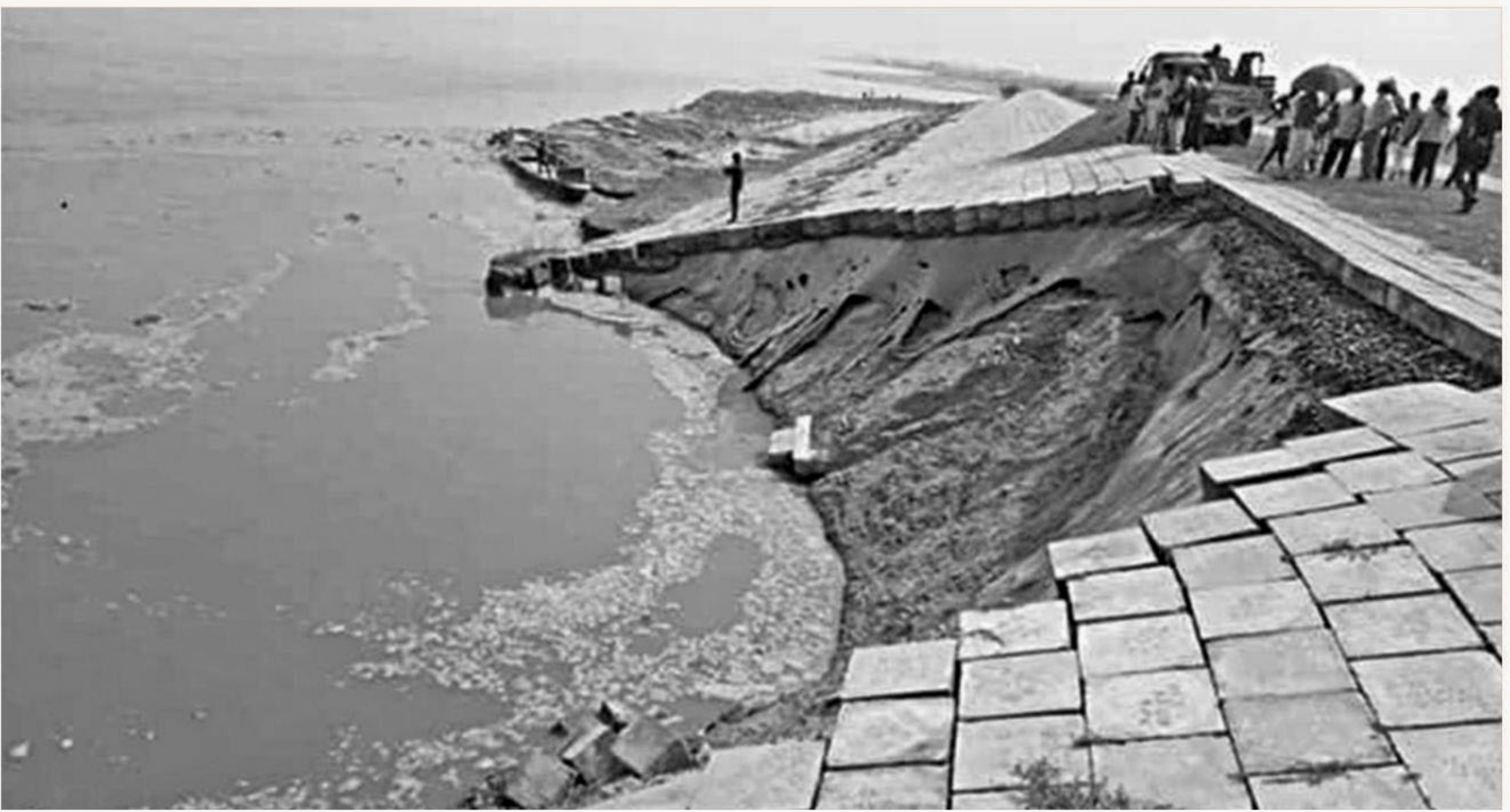
Sudden fall in water level in the Jamuna devours a portion of the crossbar, built to protect the town protection embankment, at Mollabari point in Sirajganj Sadar upazila yesterday.
