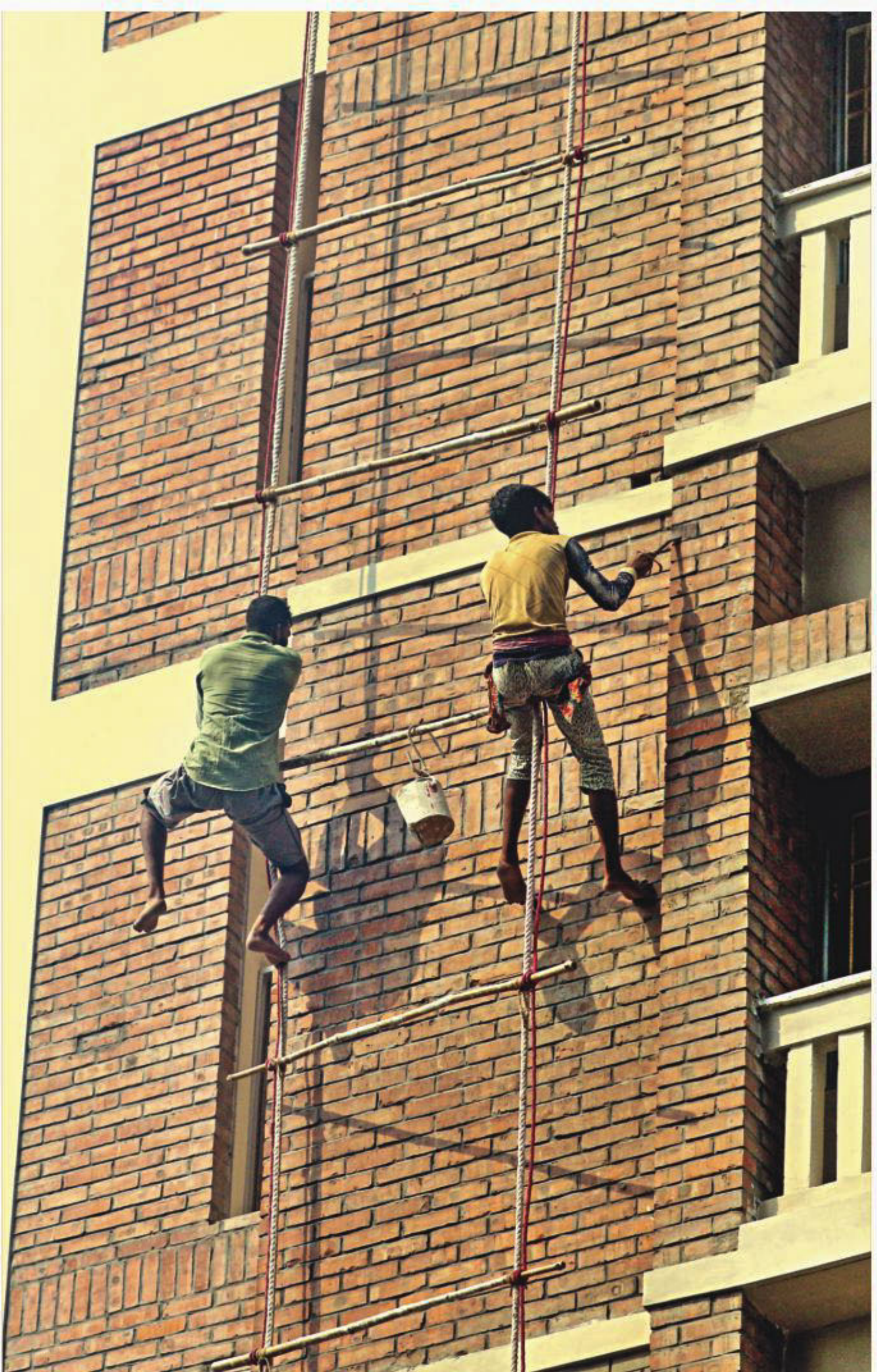
Sitting on a fragile bamboo pole, two workers plaster wall of a high-rise building on Johnson Road near Jagannath University yesterday. Construction workers often have to work without proper safety measures and in hazardous condition leading to frequent accidents.
