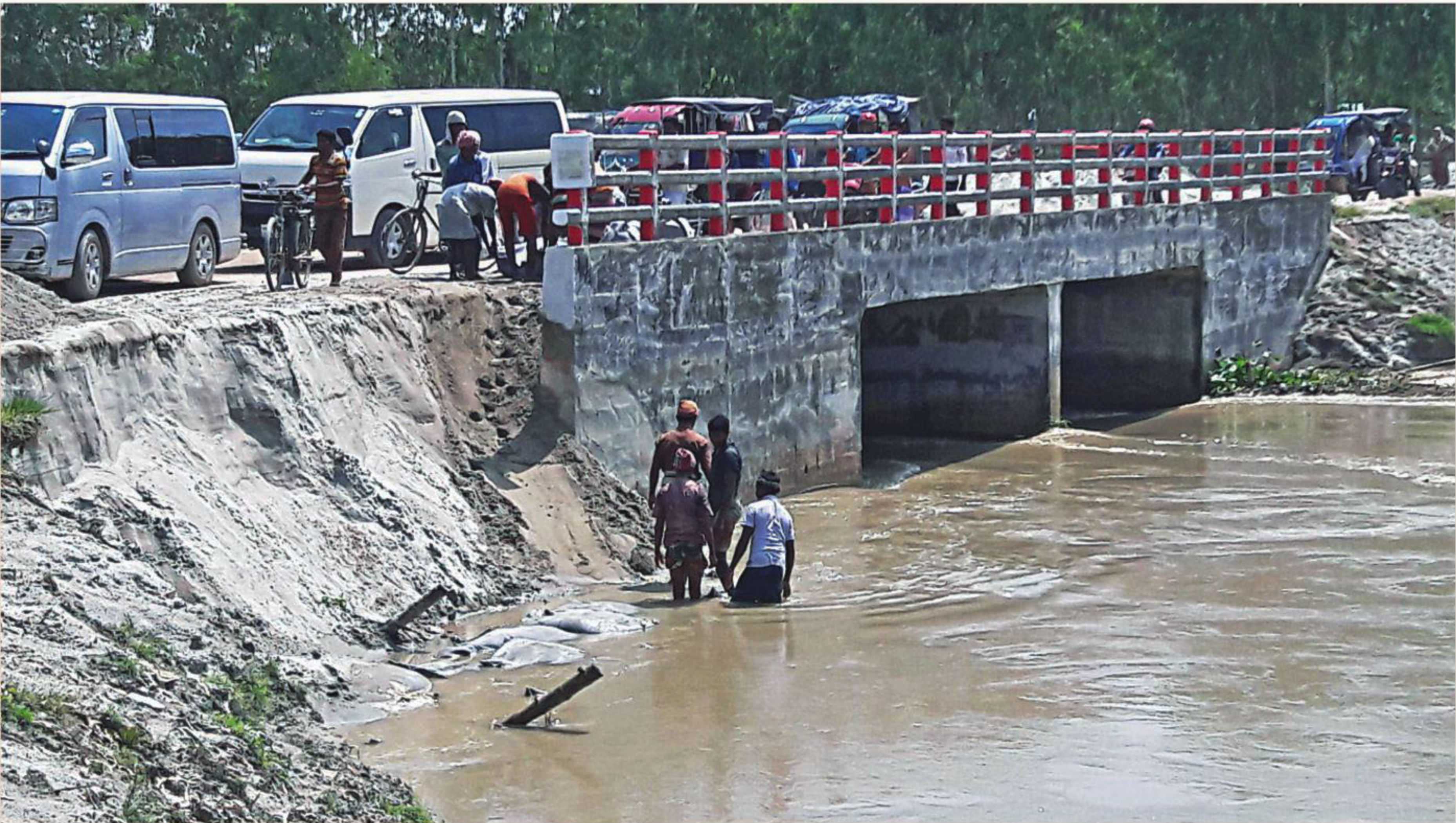
Labourers dump sandbags on an erosion-hit approach road to a culvert at Rudreshwar village in Lalmonirhat's Kaliganj upazila to protect it from erosion by the Teesta river.
