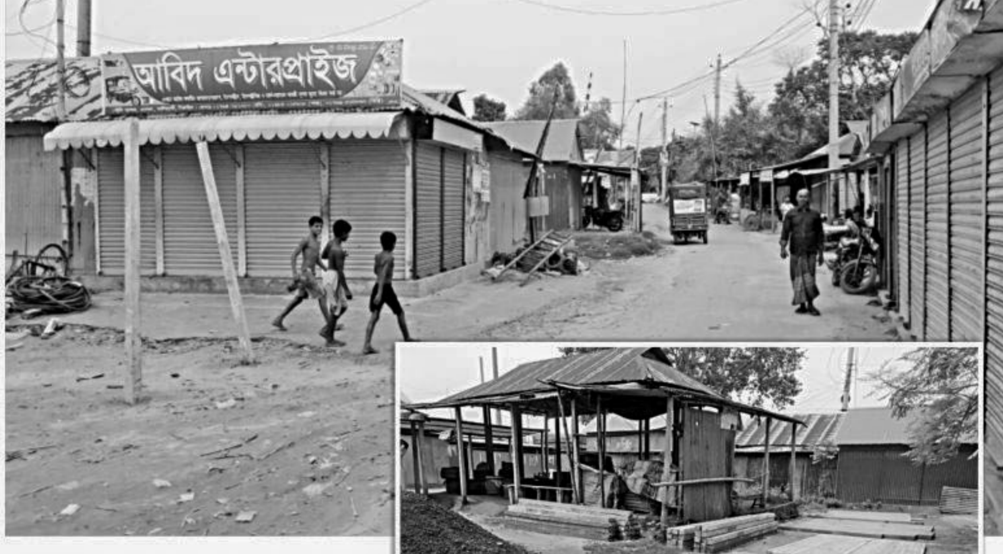
Grabbers constructed this illegal market on Roads and Highways Department land in Tangail's Kalihati upazila. Inset, ongoing construction of a shop. PHOTO: STAR
