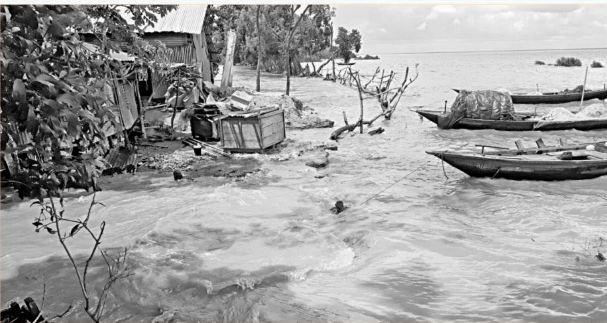
Surging tide submerges the bank of the Tentulia river following breach in the embankment in Dashmina upazila of Patuakhali. PHOTO: STAR
