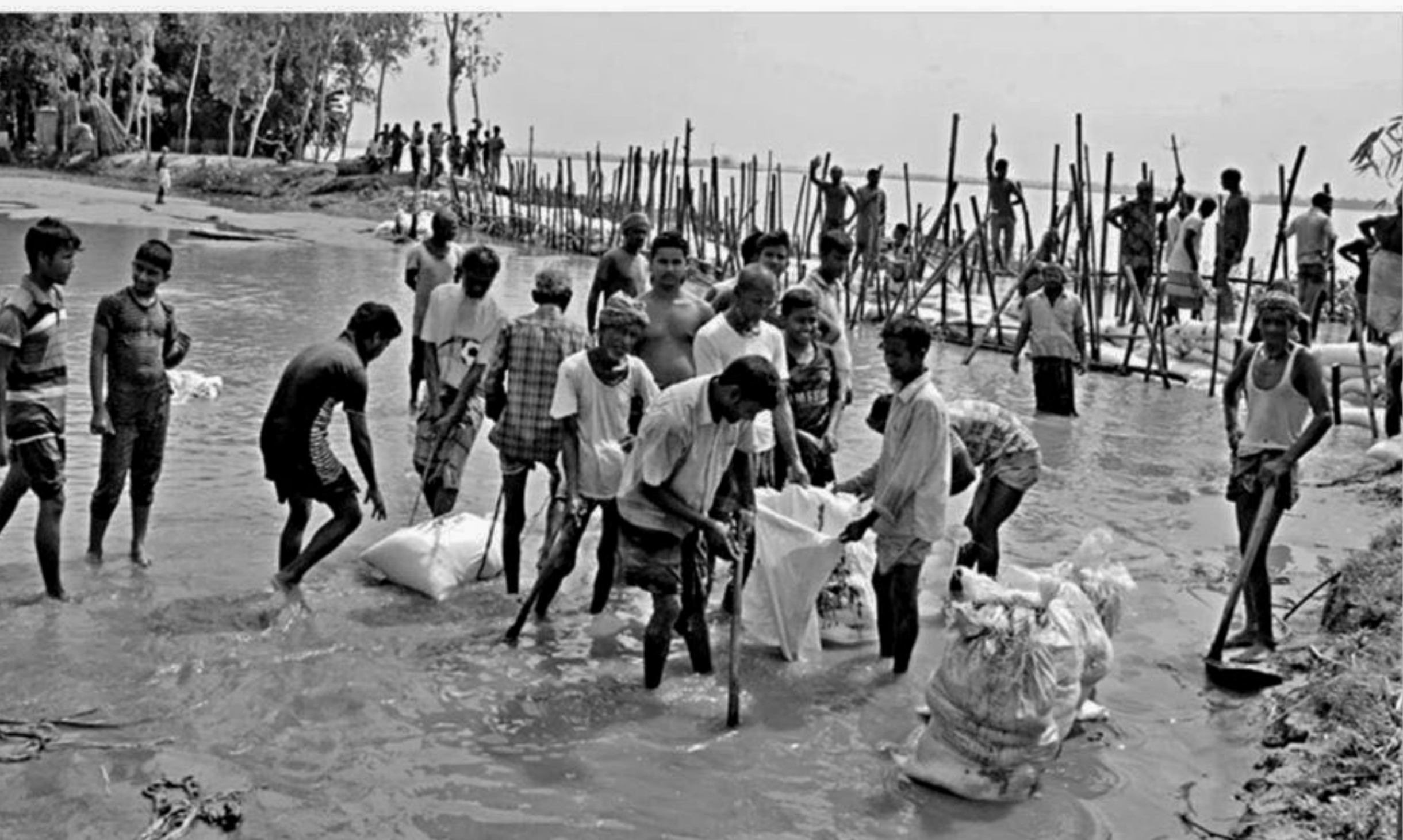
Over 100 villagers work voluntarily to rebuild a dyke that collapsed due to pressure of the Teesta water at Dhubni village in Singimari union under Hatibandha upazila of Lalmonirhat. PHOTO: STASR
