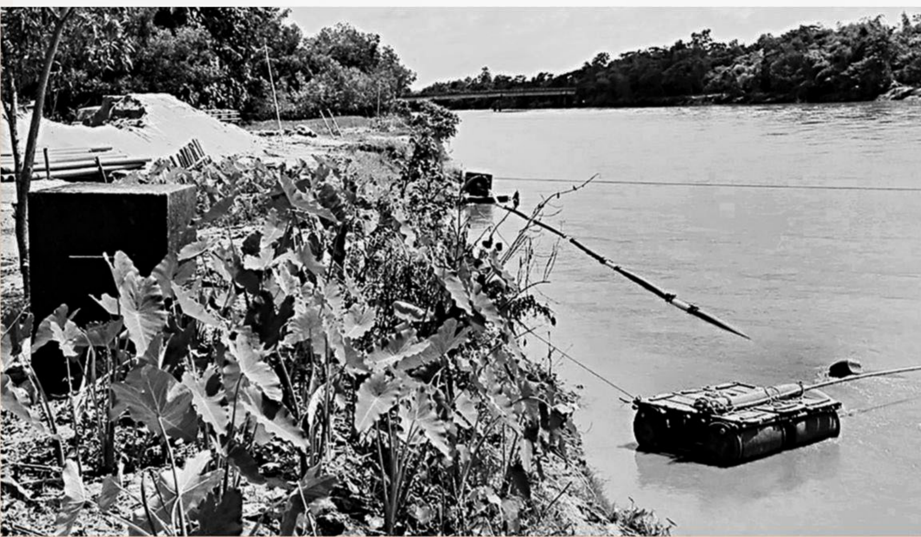
Mindless sand lifting from the Monu river poses risk to its embankment and a nearby bridge in Kulaura upazila of Moulvibazar.
