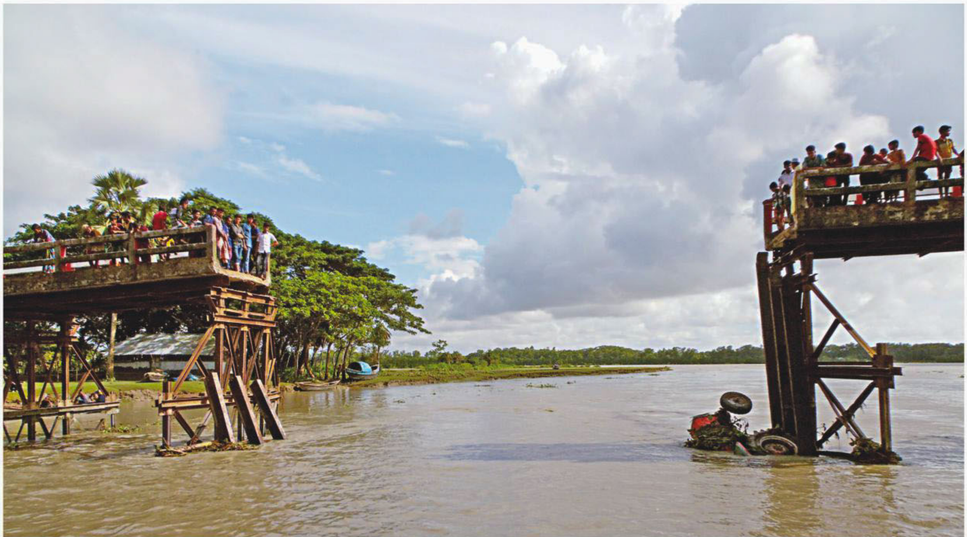
A collapsed portion of a bridge on Patuakhali's Gazalia canal under Galachipa upazila. The structure gave way when a brick-laden trailer was crossing it.
