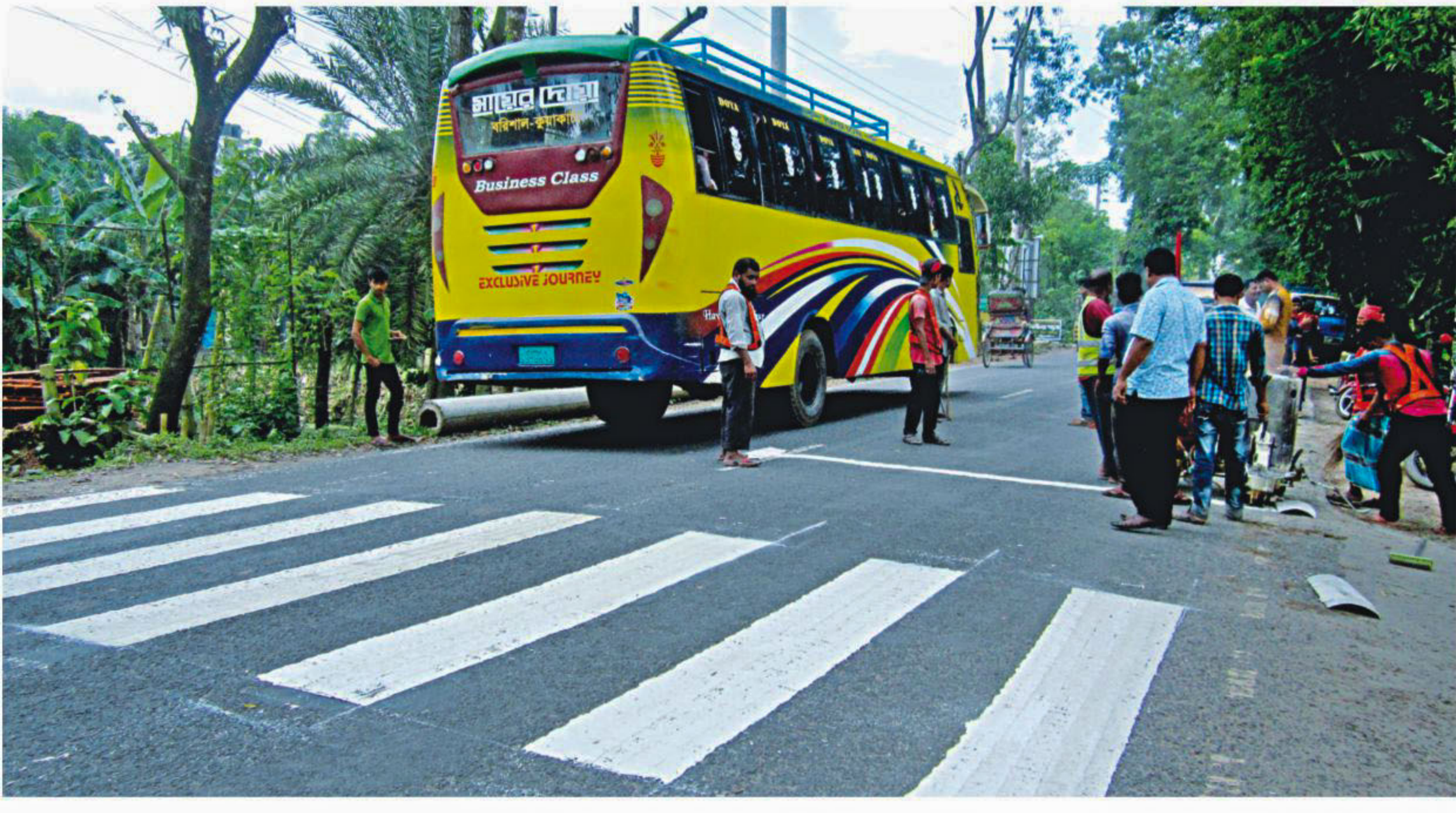
A zebra crossing is being painted on Patuakhali-Kuakata road in Patuakhali town yesterday. The authorities made the move to prevent accidents. PHOTO: STAR
