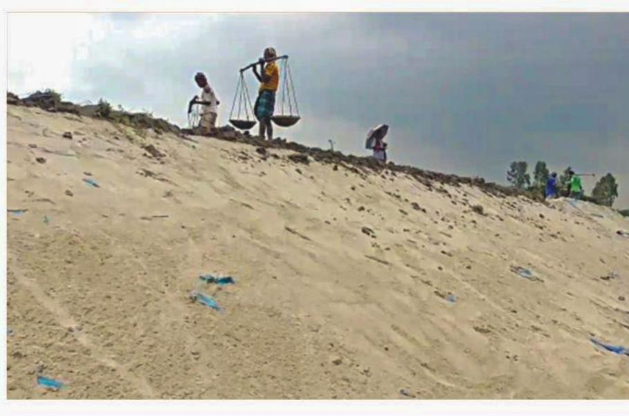
Sand extracted from the Dhepa river in Biral upazila of Dinajpur is being used to repair the flood control embankment on its bank, and right, only a thin layer of earth is put on the embankment, leaving it too weak. The Water Development Board officials said they have made the arrangement to save wastage of soil while locals have expressed worry about possible erosion and collapse of the embankment even during an average flood. PHOTO: STAR
