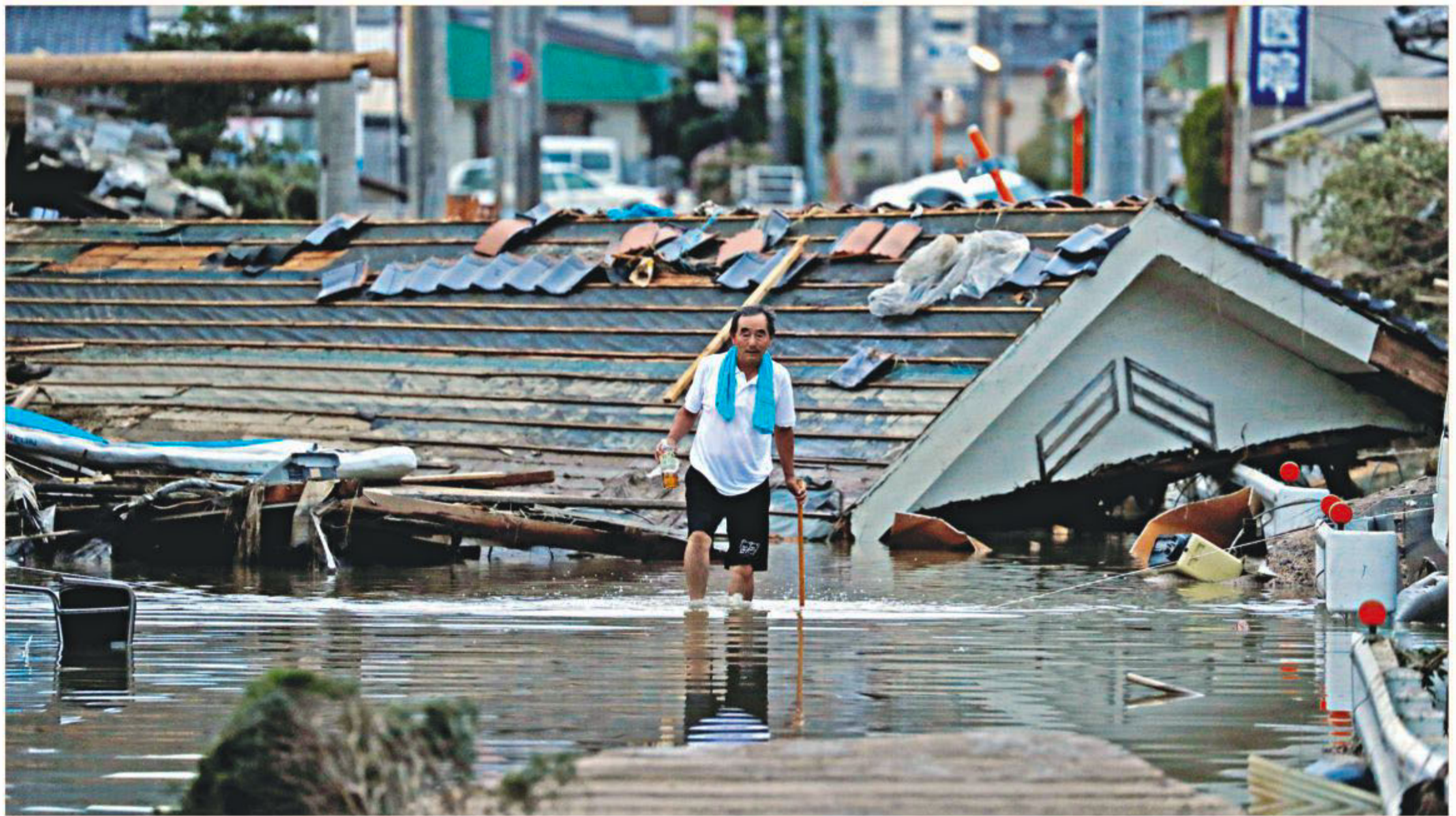
A local resident walks in front of submerged and destroyed houses in a flooded area in Mabi town in Kurashiki, Okayama Prefecture, Japan, yesterday. The death toll from torrential rain and landslides in western Japan rose to 81 people yesterday. PHOTO: REUTERS
