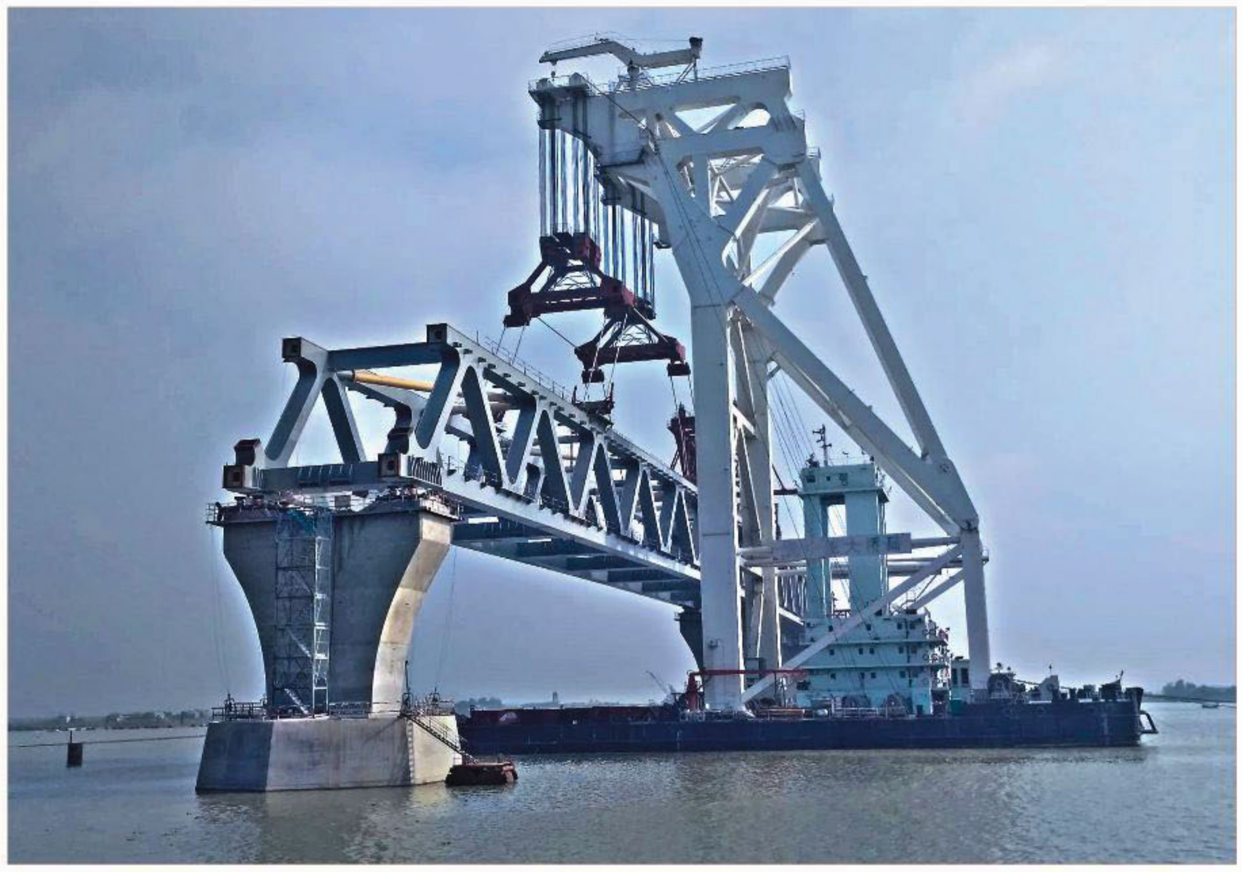
This photo taken on May 13 shows the fourth span of the Padma Bridge being installed between pillars 40 and 41 on the Jazira side. The cost of the project is going to increase again as the government plans to acquire additional land for Tk 1,400 crore.
