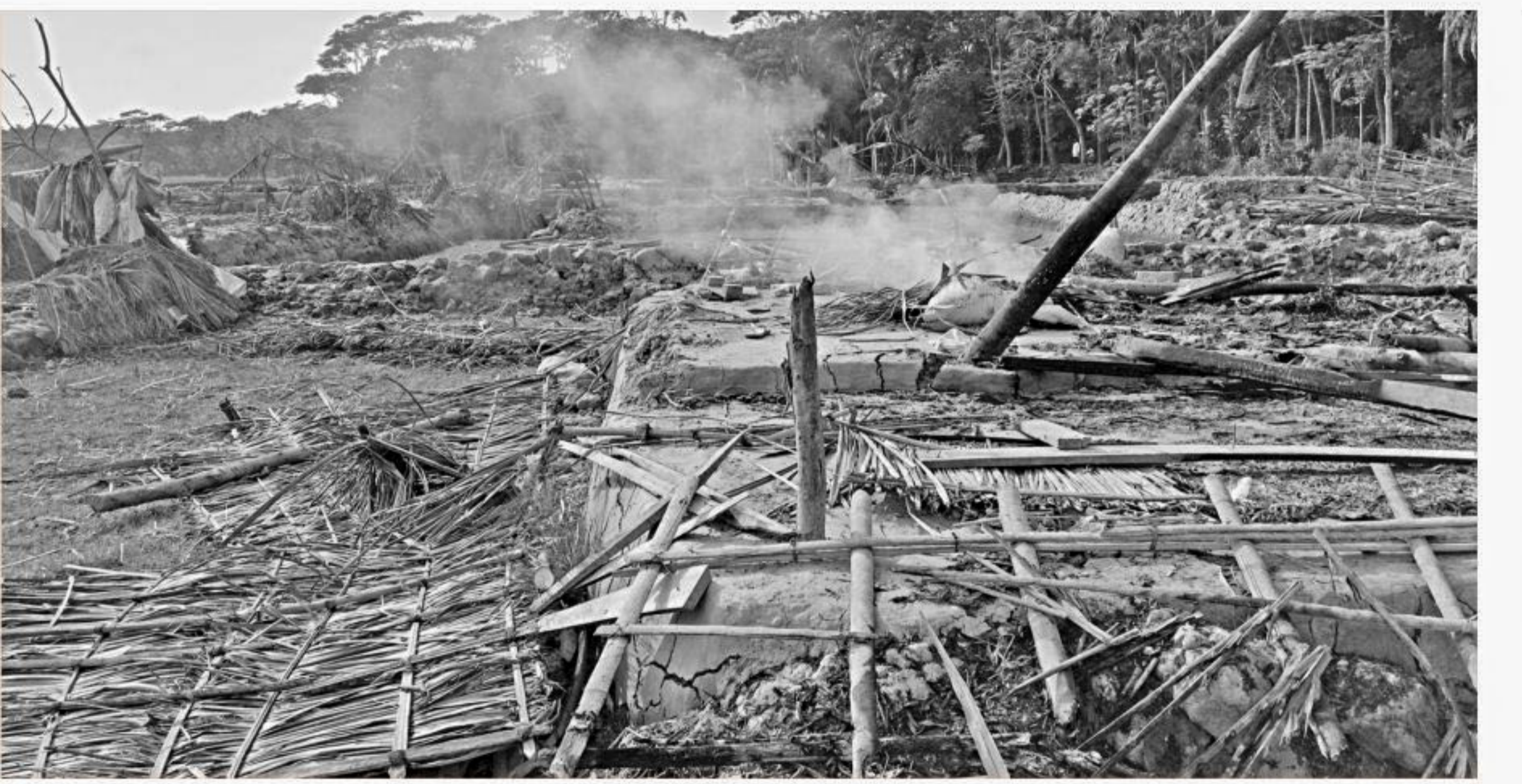
Charred remains of shanties at Dakkhin Badhal village in Sharankhola upazila of Bagerhat after criminals set fire to the structures belonging to landless people on Saturday. PHOTO: STAR
