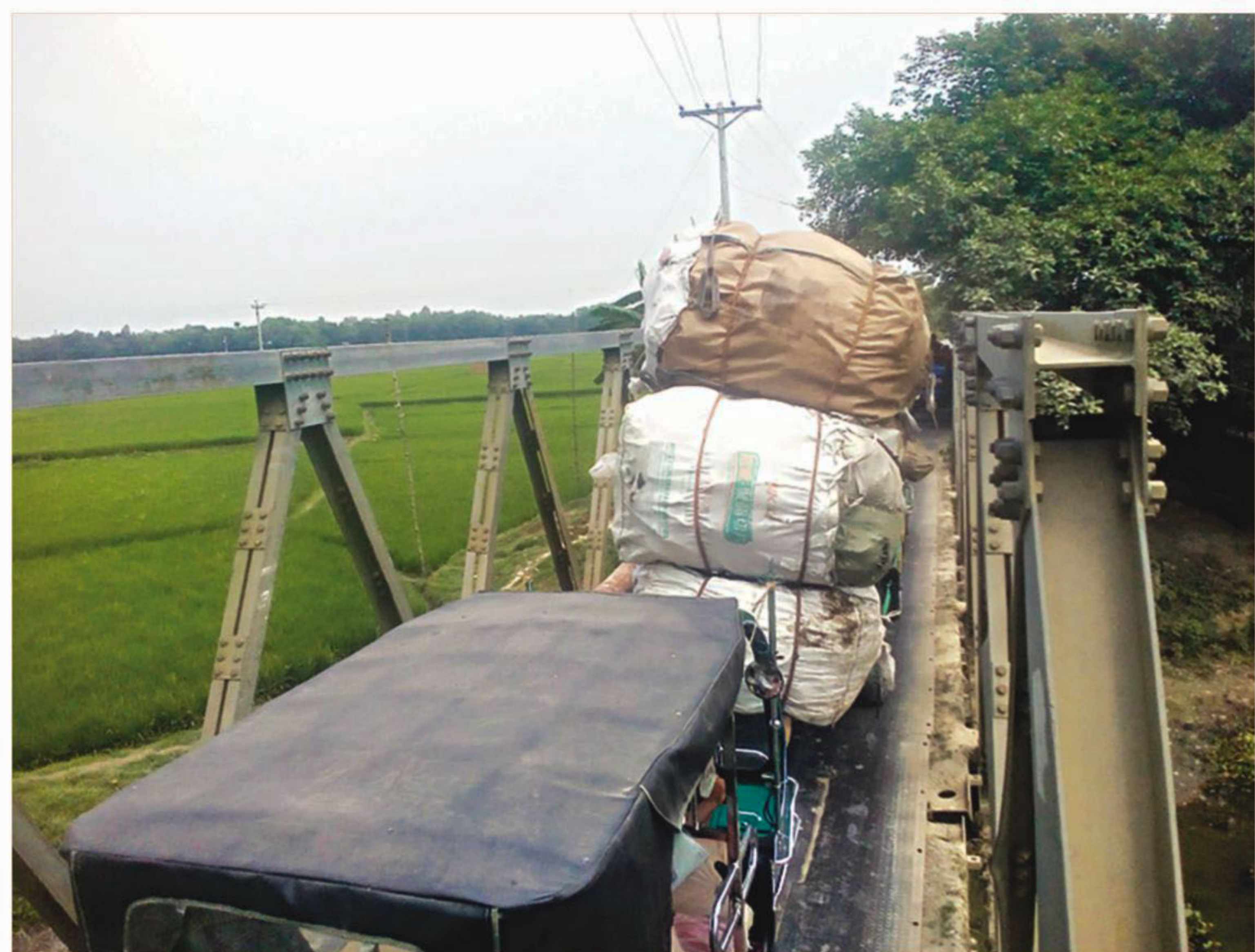
The scene at a Bailey bridge in Nagarpur upazila of Tangail.
