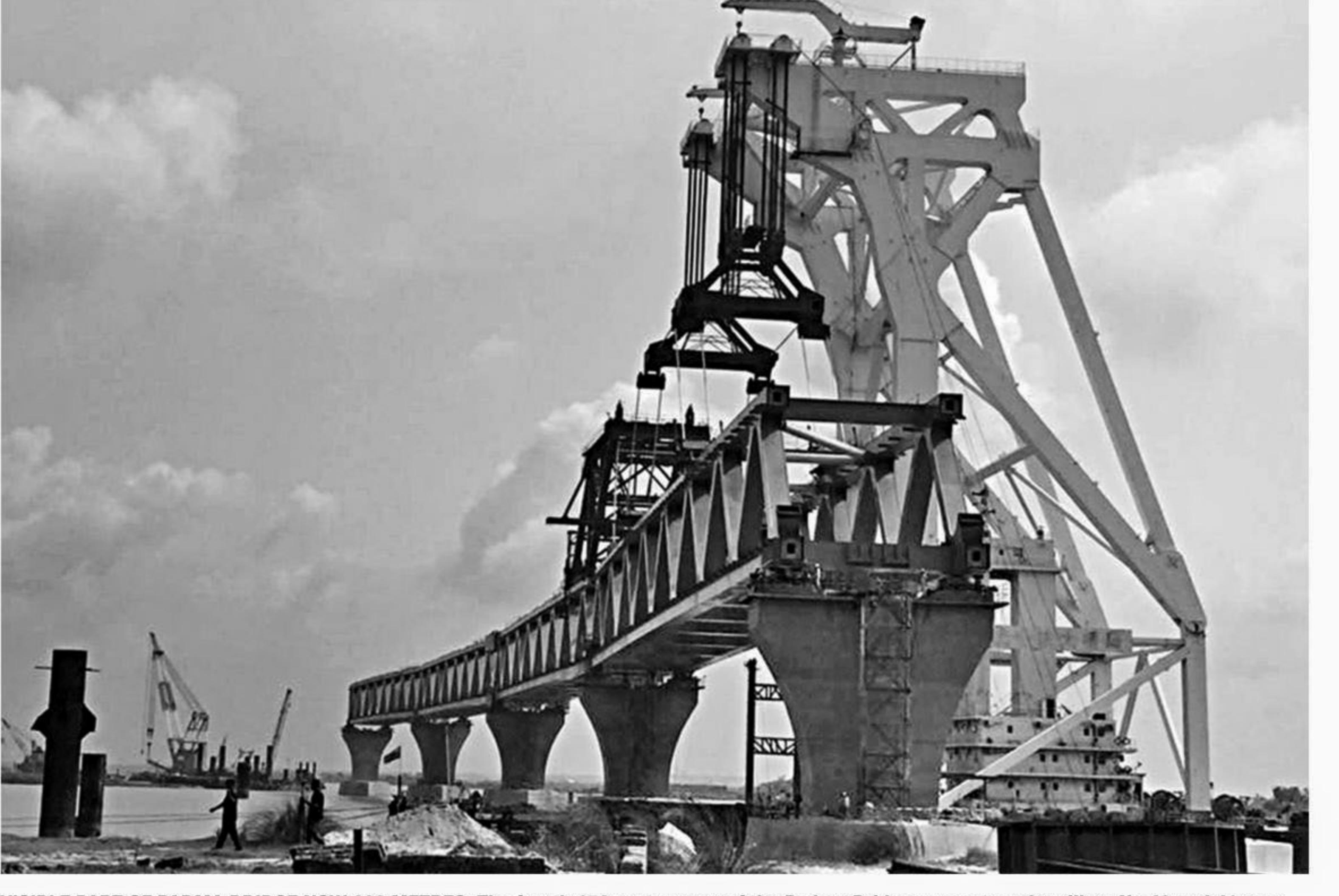
**VISIBLE PART OF PADMA BRIDGE NOW 600 METRES:** The fourth 150-metre span of the Padma Bridge was set on the pillars No 40 and 41 near its Jazira end in Shariatpur yesterday, making visible 600-metre structure of the under-construction bridge across the mighty Padma. When completed, the 6.15 kilometre-long bridge will ease communication between the country's southern region and the capital.
