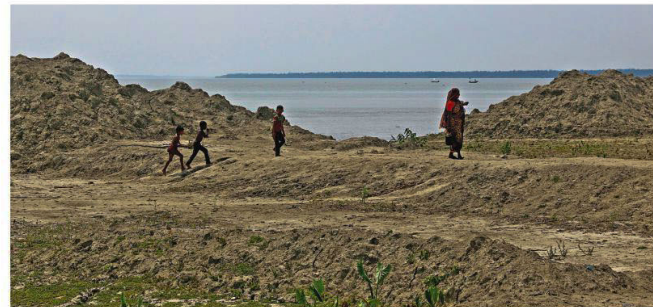
These eroding earthen mounds are some of the few remnants of the embankment ruined by cyclones and river erosion.
