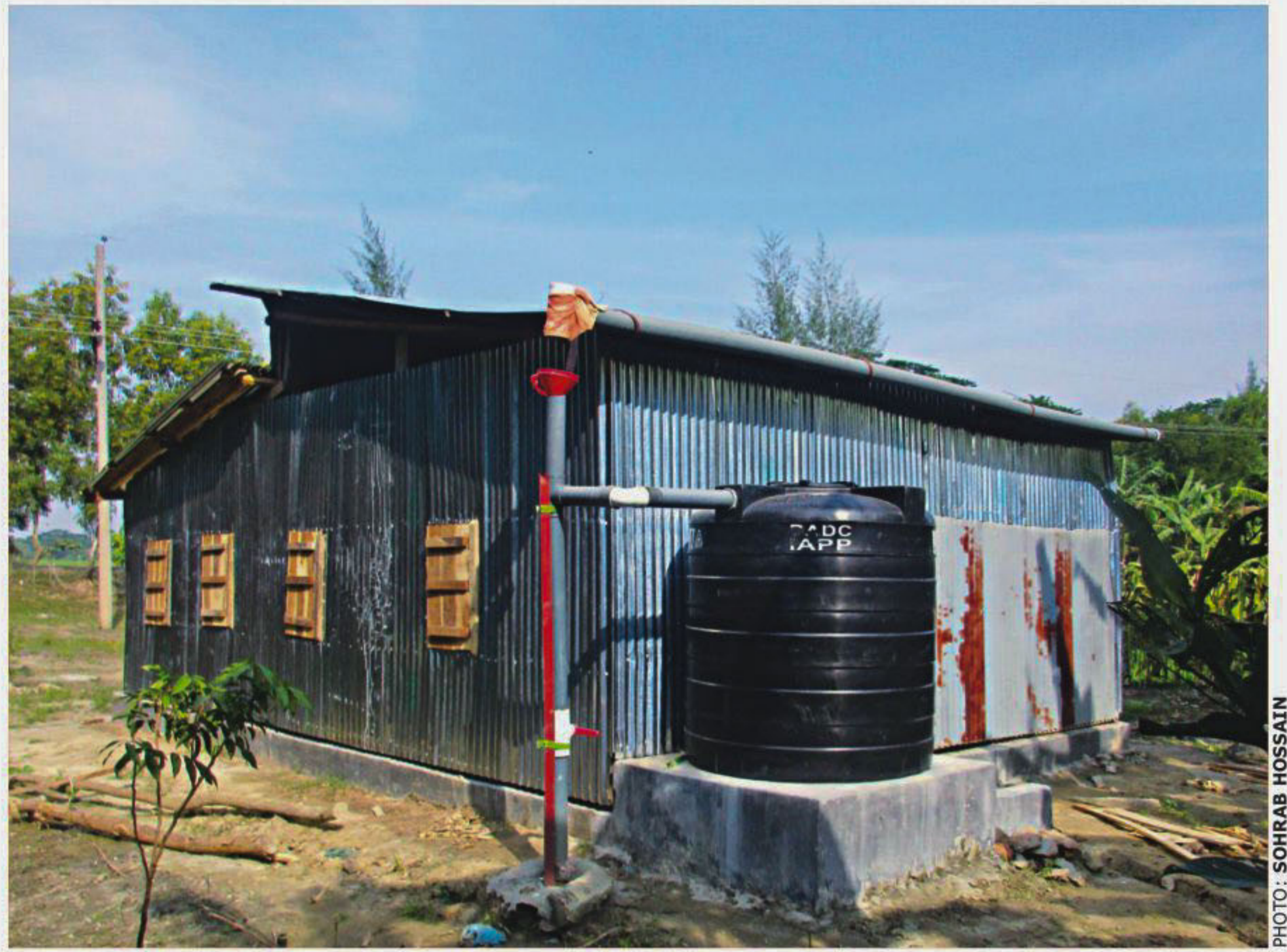
A rainwater harvesting plant at Latachalee under Kalapara upazila in Patuakhali.
