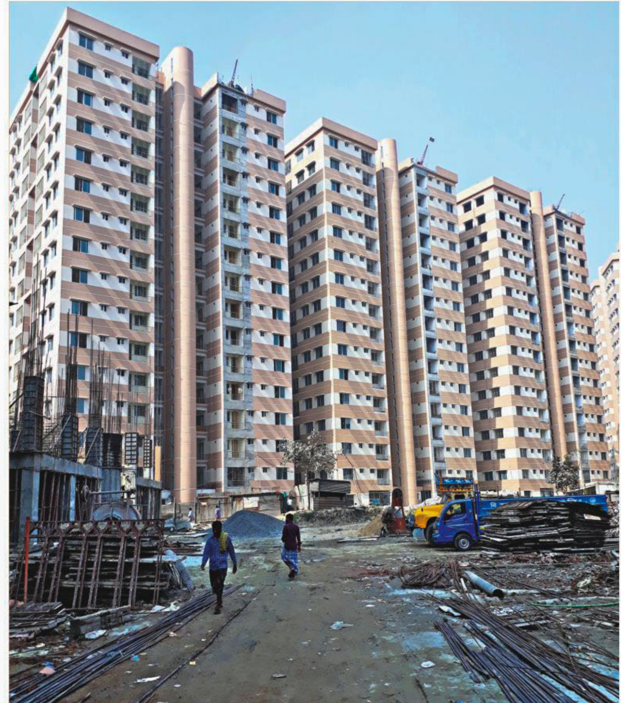
The buildings under construction. The photo was taken recently.
