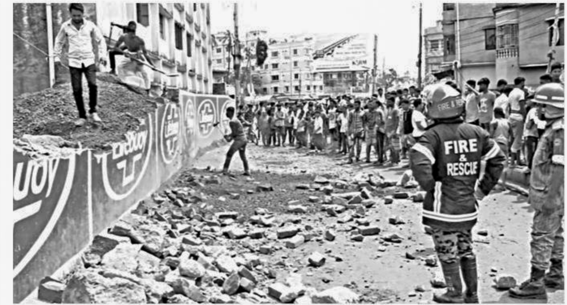
A part of the boundary wall of Shibrampur Model Government Primary School in Pabna town collapses yesterday, killing a student and injuring three others. PHOTO: STAR
