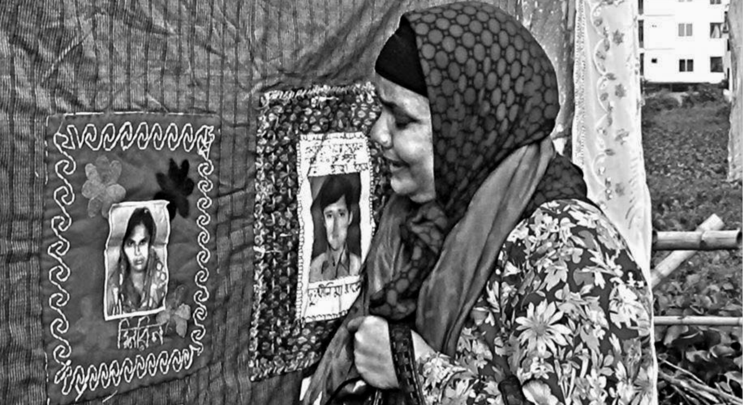
Rahela Khatun, mother of Rana Plaza collapse victim Rabbi, cries near the portrait of her son at an exhibition in front of the site in Savar yesterday. It was organised in memory of the people killed and injured in the nine-storey building collapse on April 24, 2013. More than 1,100 people, most of them garment workers, lost their lives in the tragedy. Bangladesh Garment Sramik Sanghati hosted the exhibition titled "Smriti Katha o Kotha" (Memories on quilts and in words), featuring quilts bearing the photographs of the victims. The quilts were designed by families of the deceased and survivors. Marking the fifth anniversary of the tragedy, photographer Taslima Akhter and American artist Robin Barson planned the event with the theme, "Remember the dead, fight for the living".
