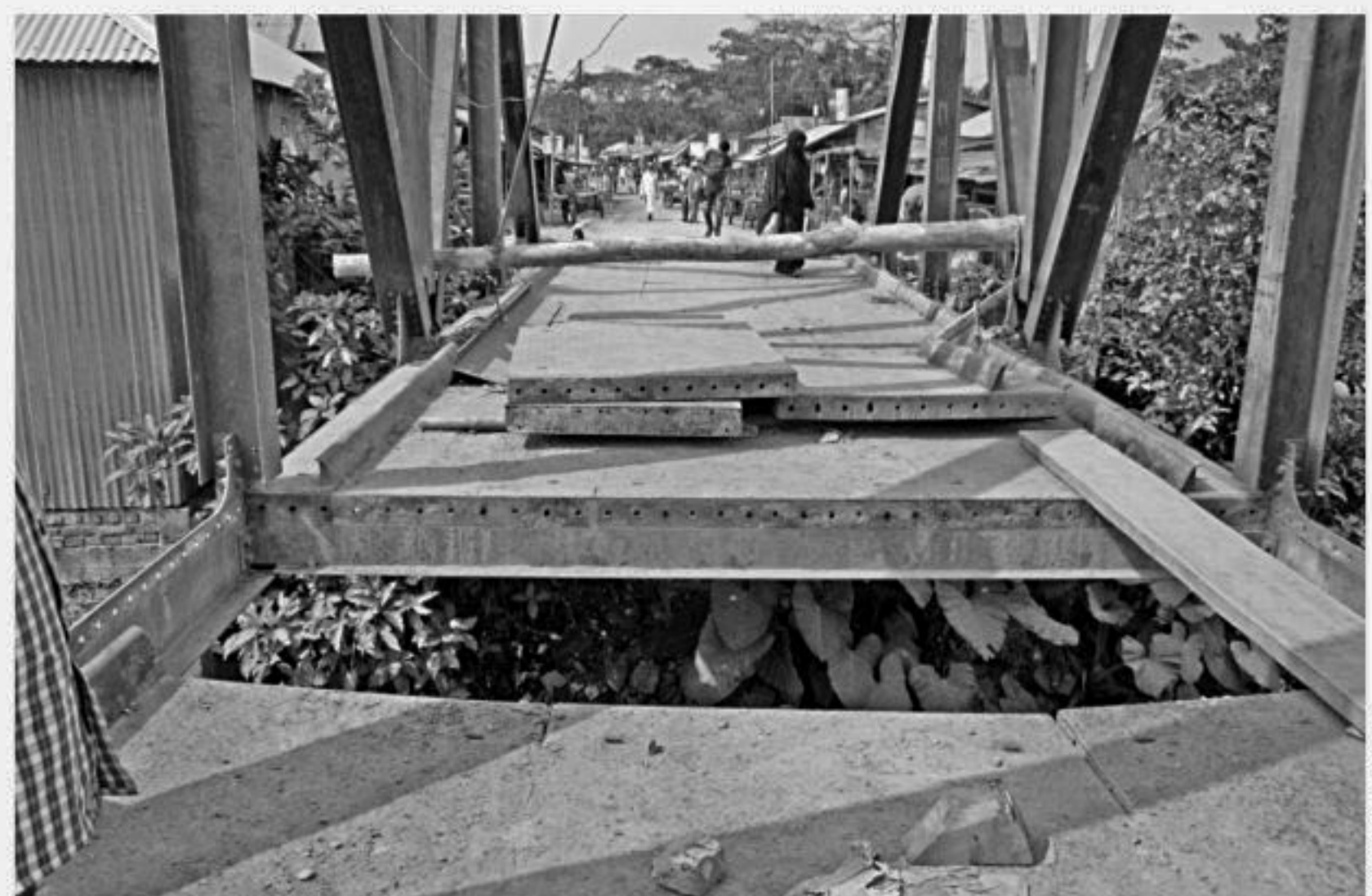
A Bailey bridge over Arpangashia canal lying damaged for the last eight days in Amtali upazila of Barguna. The photo was taken a few days ago.
