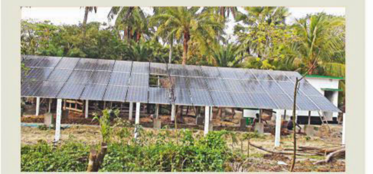
SOLAR-POWERED IRRIGATION: Bangladesh Agriculture Development Corporation is successfully using this solar panel to draw water for irrigating Boro fields at Pashchim Baniary village in Matibhanga union under Nazirpur upazila of Pirojpur. The first of its kind initiative to provide low-cost irrigation has drawn appreciation from local farmers. PHOTO: STAR
