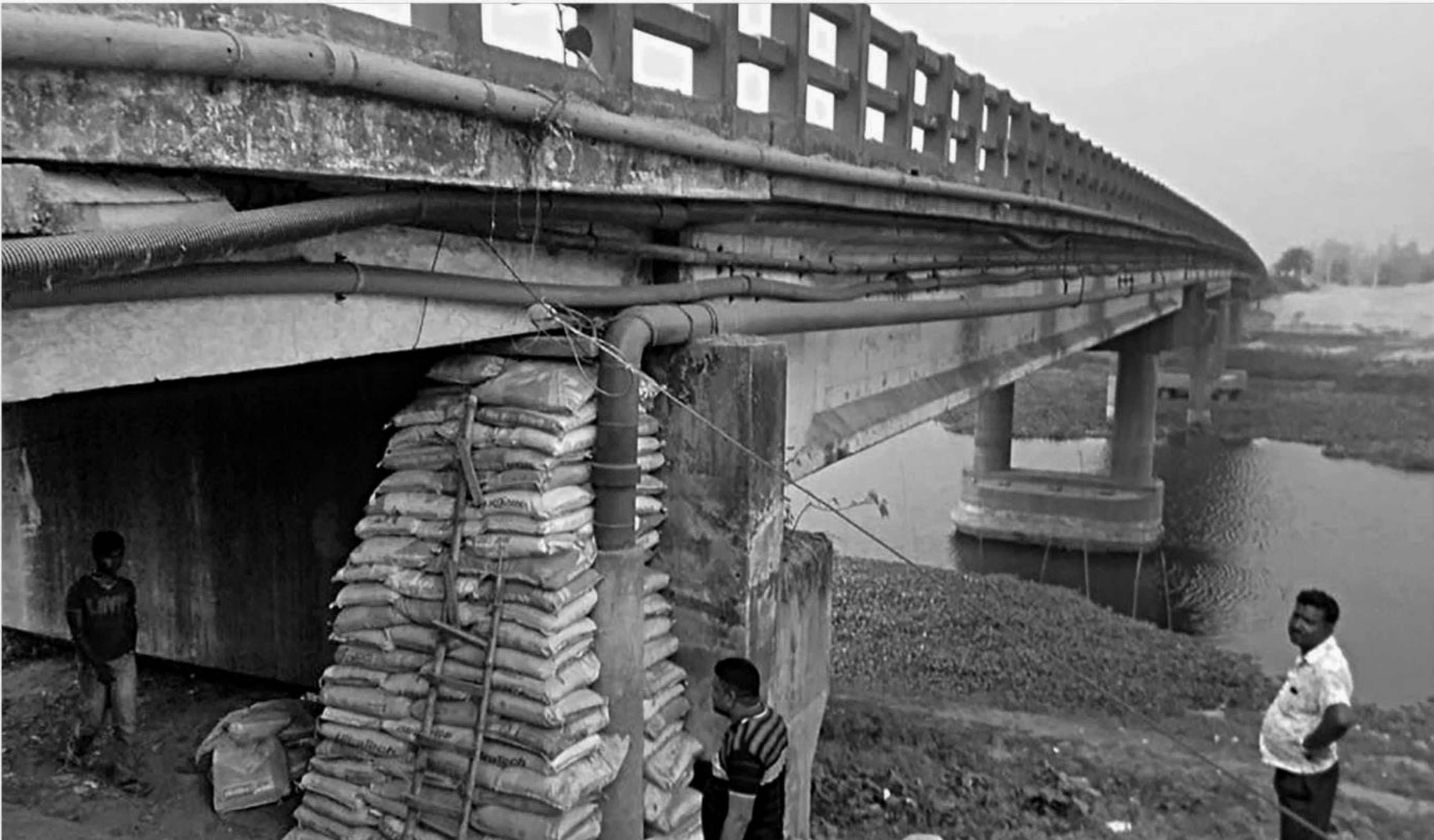
Sandbags are set to protect an affected pillar of Nolkha Bridge near Bangabandhu Multipurpose Bridge in Sirajganj. Below, a bamboo bridge over Kalikura canal is lying unused after damage of its approach roads during last year's flood in Kaliganj upazila of Lalmonirhat and a bridge over the Ratnai river on Lalmonirhat-Mogholhat road in Lalmonirhat Sadar upazila's Durakuti area faces risk as three of its four girders are vulnerable.
