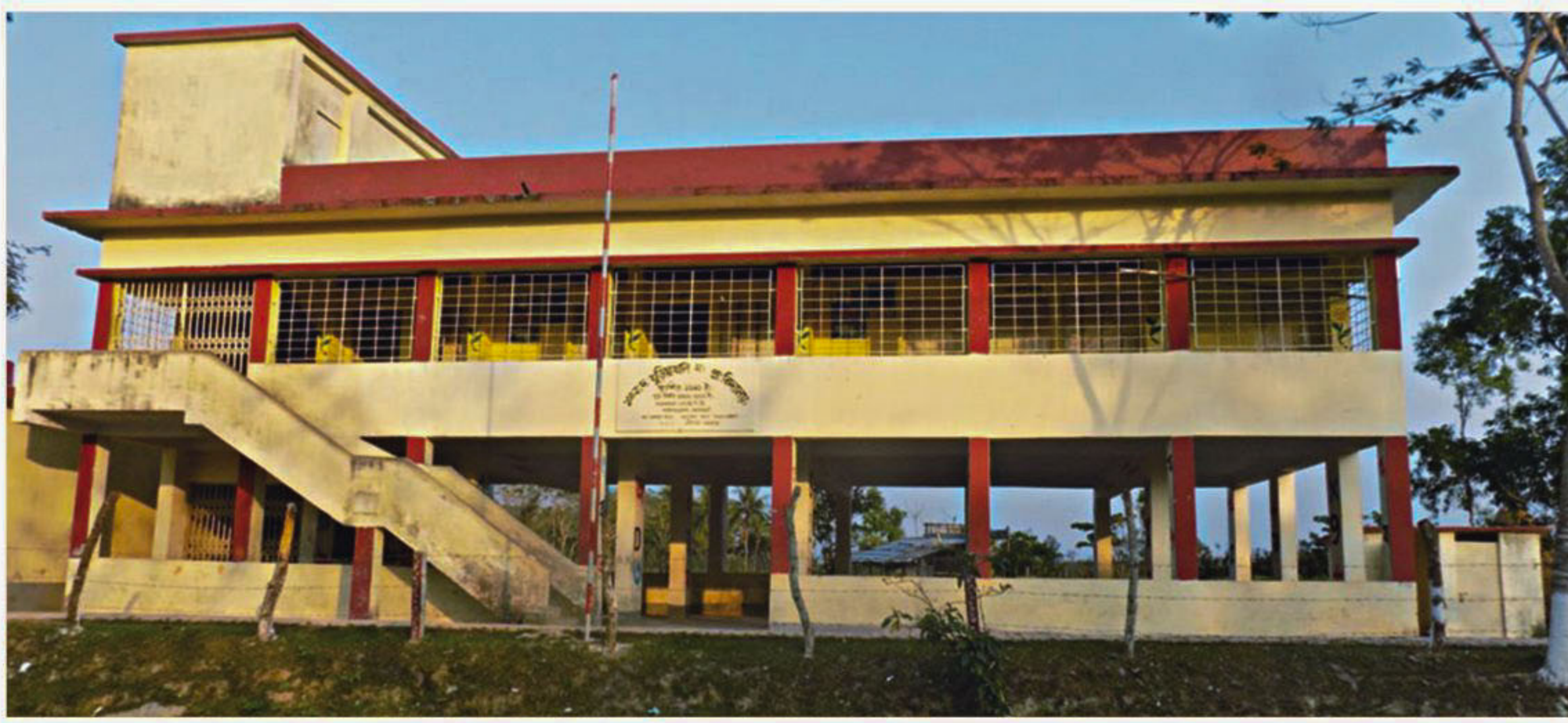
Khaulia Government Primary School, a school-cum-cyclone shelter in Morelganj upazila of Bagerhat.
