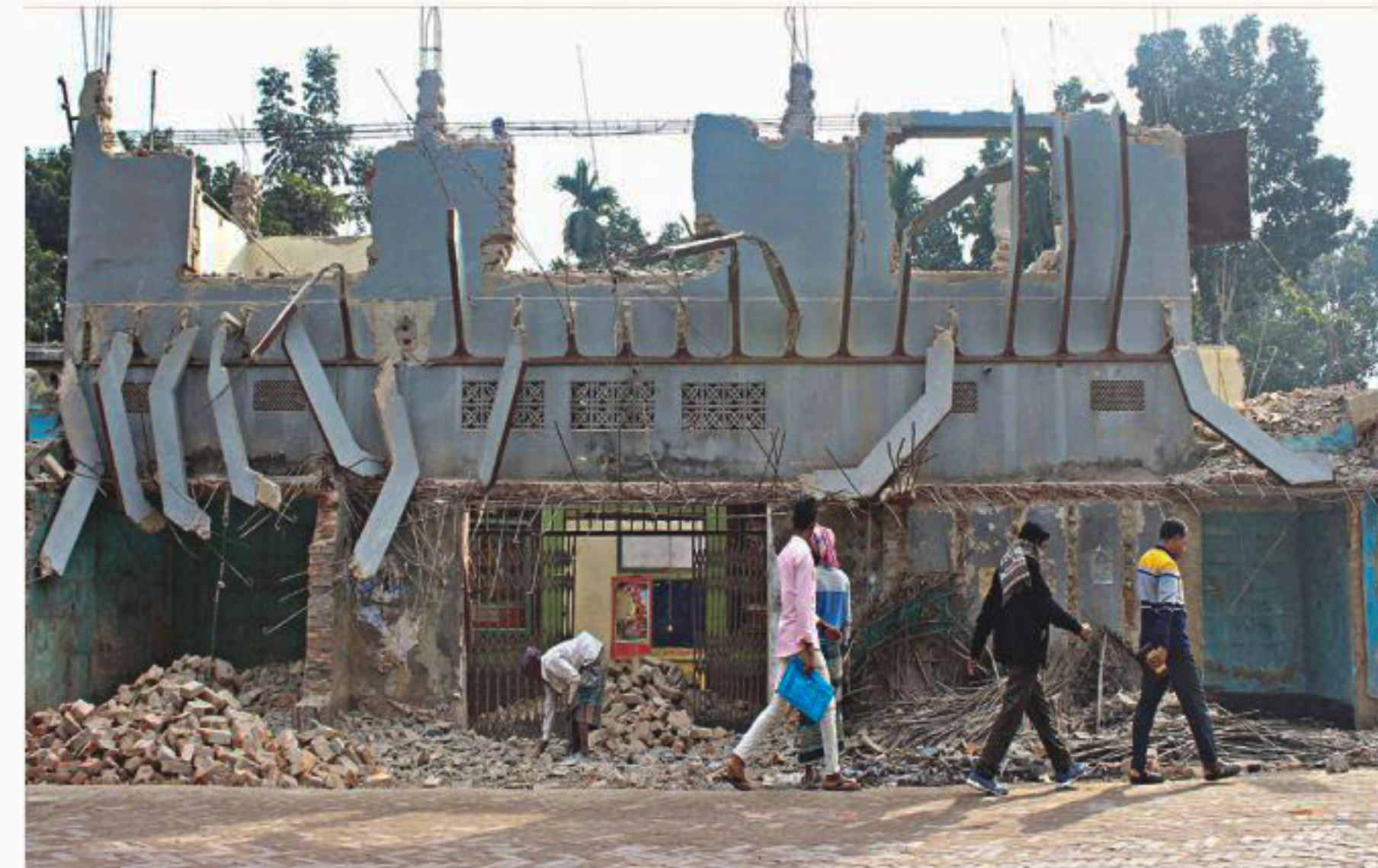
Demolition underway of Rajbari's largest cinema hall at Boropul.
