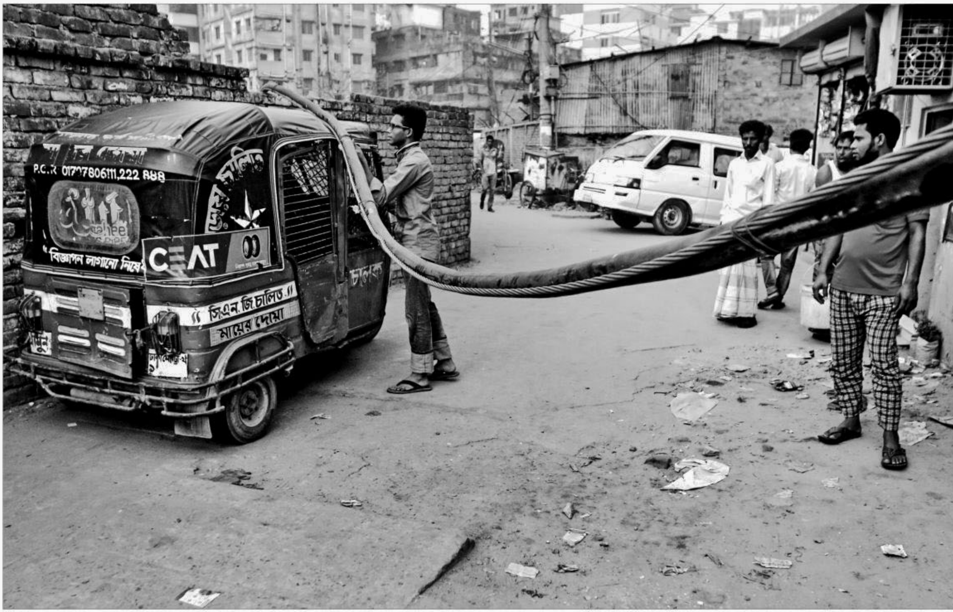
A youth holds up a high-tension electric cable to let an auto-rickshaw pass under it on a street in the capital's Mohakhali. Several electric poles and a transformer in the vicinity were damaged early yesterday morning when an overhead high-tension cable running across the road was entangled on the top of a cargo vehicle on the nearby Shaheed Tajuddin Ahmad Sarani. No safety measures were visible at the spot to protect citizens from possible electrical accident when this photo was taken around 10:00am.
