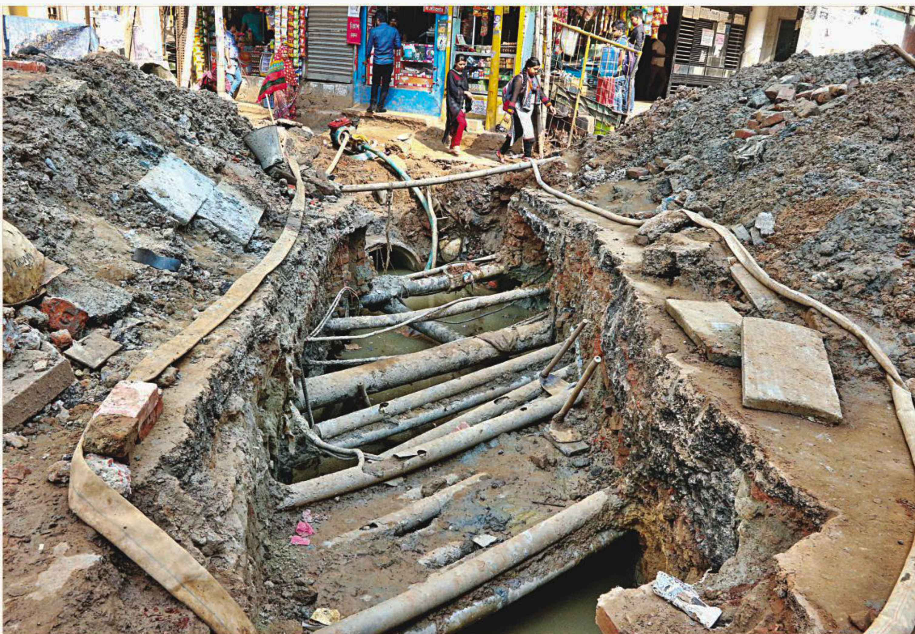
Crisscrossing utility lines under a dug up road in the capital's Moghbazar. Dhaka North City Corporation has been working for the last two months to install a large concrete pipe under the road to upgrade the sewer in the area. However, the officials came upon these utility connections while trying to connect the large pipe to the city's main sewer system. The photo was taken recently.
