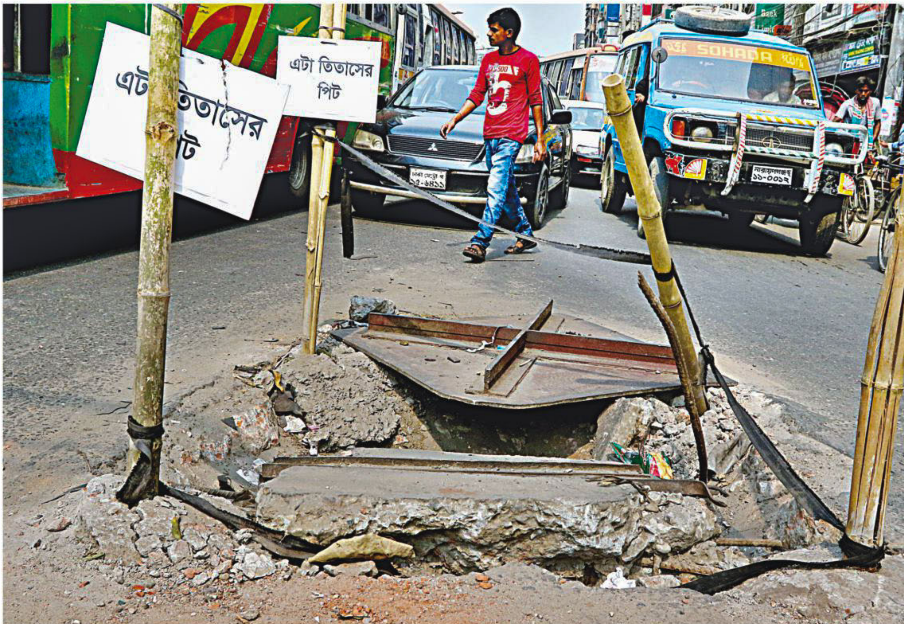
The covers for an underground junction of Titas gas lines lie broken on this Old Dhaka road for several months. With no steps from the authorities, some local traders on their own demarcated the point with bamboo poles. To alert people, they also hung signs reading, "This is a pit of Titas". The photo was taken at Tanti Bazar on Thursday.
