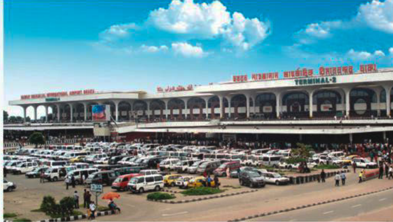
Passenger Terminal Building at Hazrat Shahjalal International Airport
