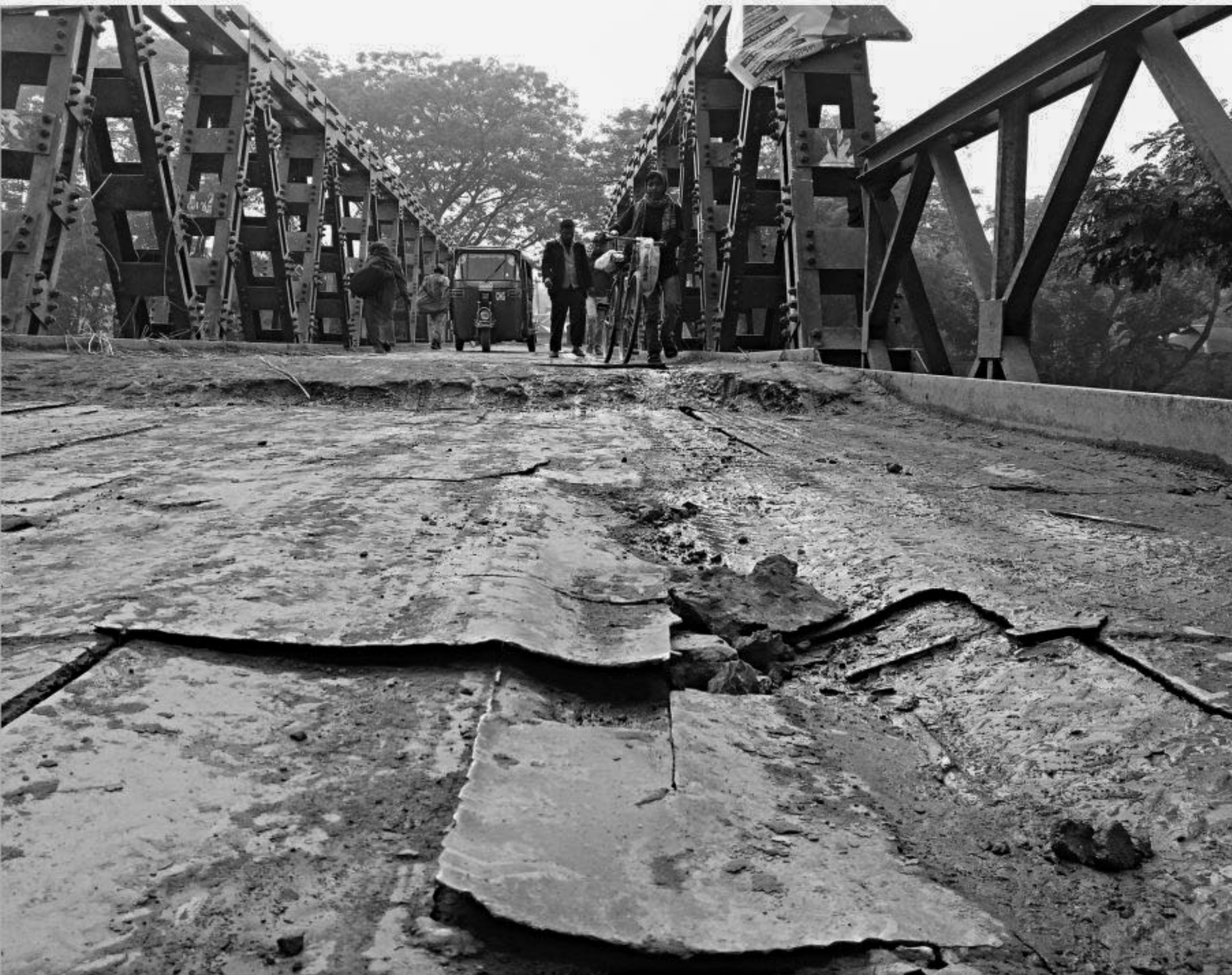
A Bailey bridge lies in an awful state for years in Mymensingh's Trishal upazila.
