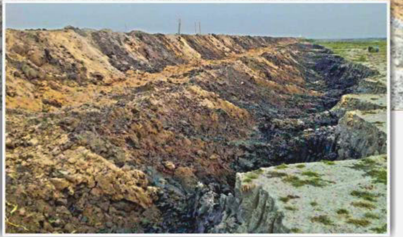
An embankment being built on Thal haor (water body) in Chandrasona under Dharmapasha upazila in Sunamganj district. There is a rule that earth has to be collected from a place at least 100-metre away from the site. However, the earth is being collected digging the land right along the dyke (inset), weakening the very structure. The photo was taken recently.
