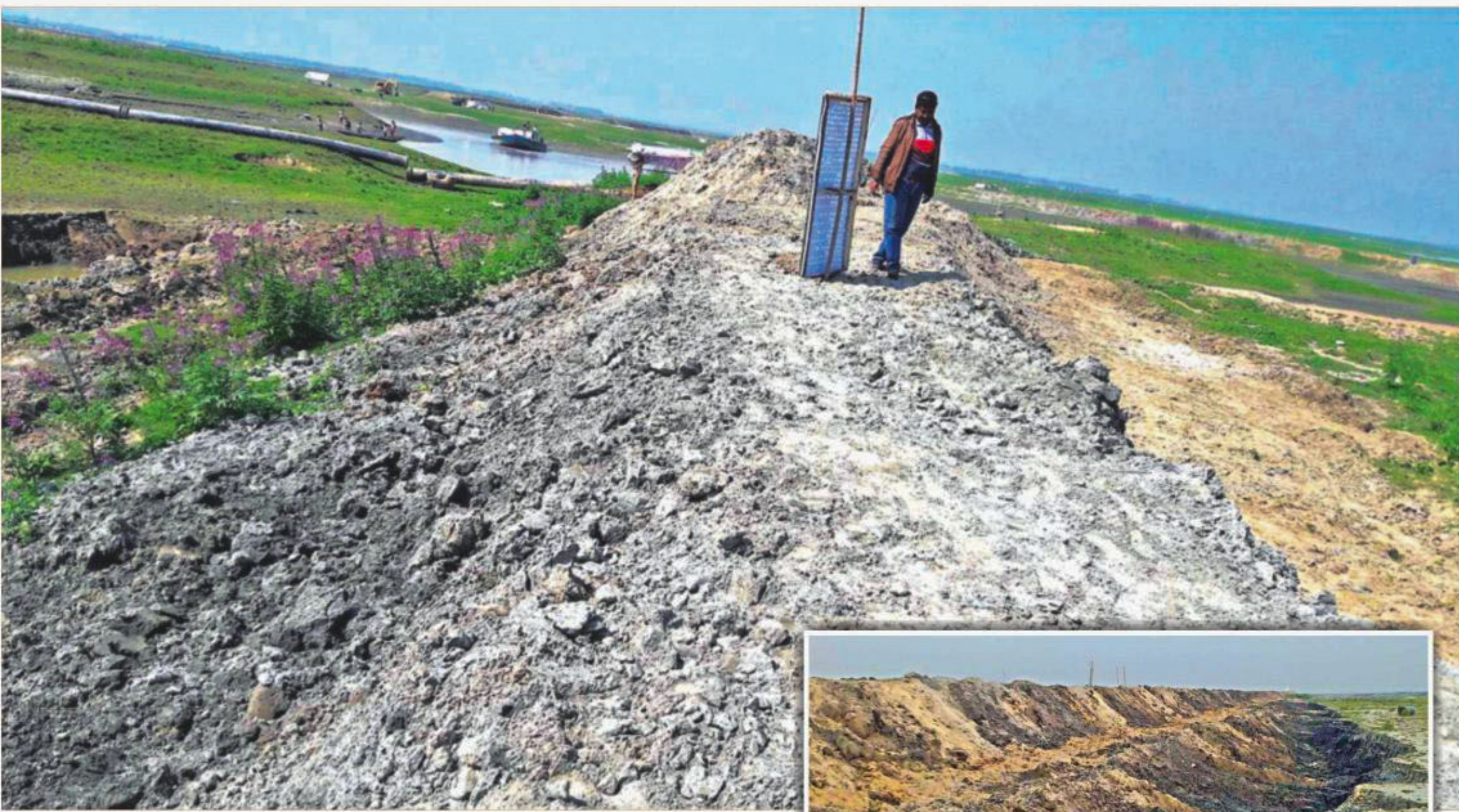
An embankment being built on Thal haor (water body) in Chandrasona under Dharmapasha upazila in Sunamganj district. There is a rule that earth has to be collected from a place at least 100-metre away from the site. However, the earth is being collected digging the land right along the dyke (inset), weakening the very structure. The photo was taken recently.
