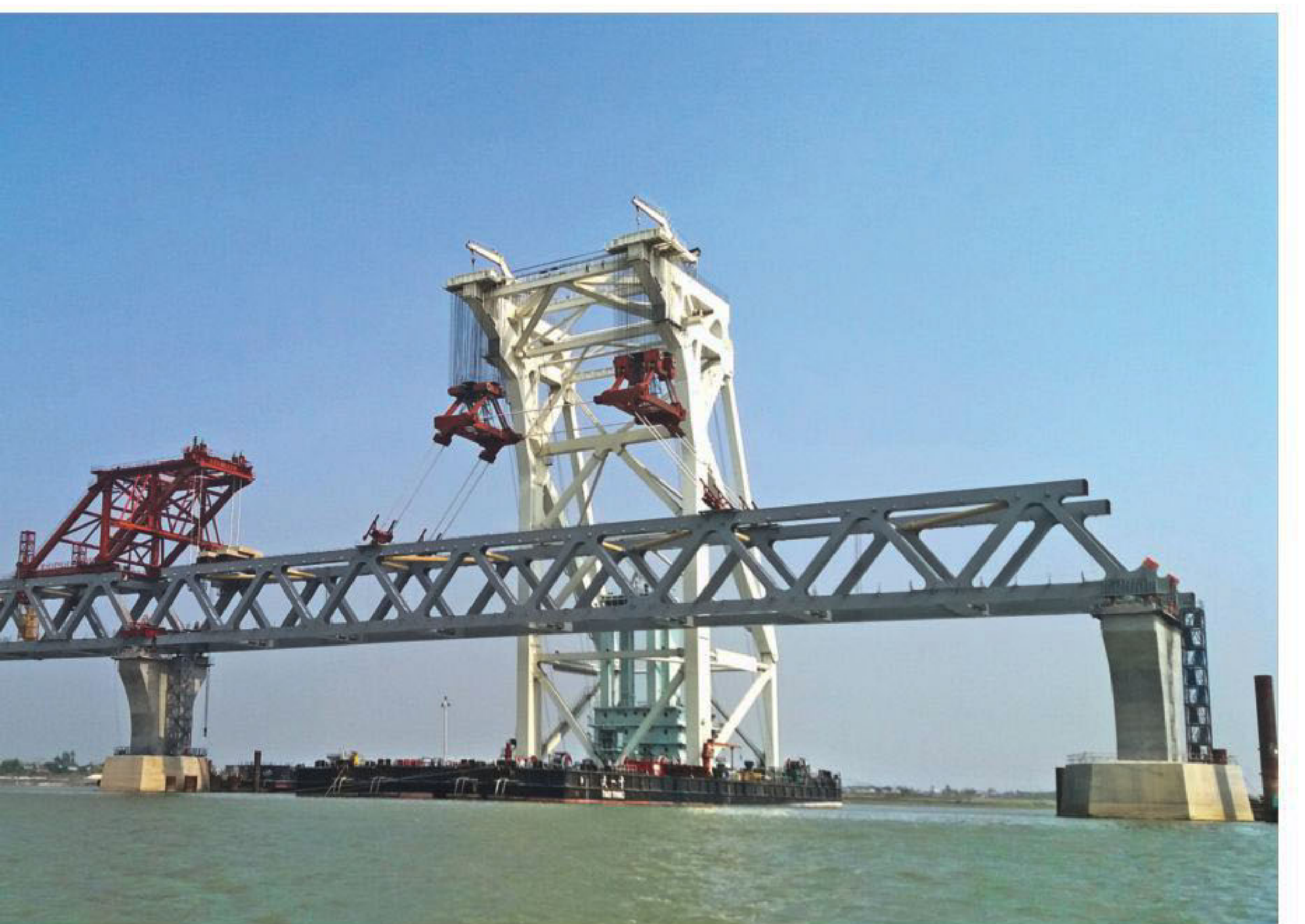
A floating crane sets the second span atop a set of piers of the Padma Bridge yesterday. With the second superstructure installed, 300 metres of the much-awaited bridge is now visible. The bridge is scheduled to be completed by December this year.
