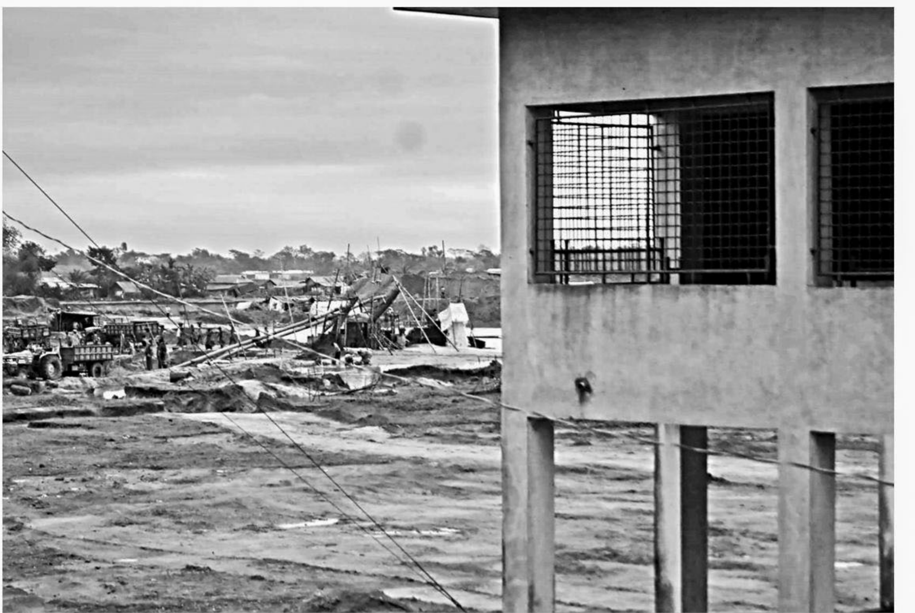
TOO GREEDY, TOO CALLOUS: Illegal stone extractors have dug large holes just beside Kalairag Government Primary School in Companyganj upazila of Sylhet, posing landslide risk for the school and nearby dwellings.
